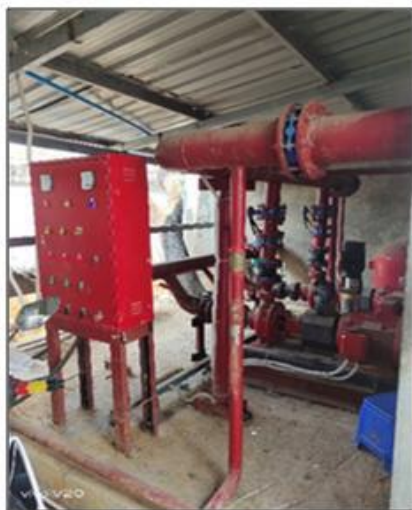
Figure 0-9: Fire Fighting System Equipment
