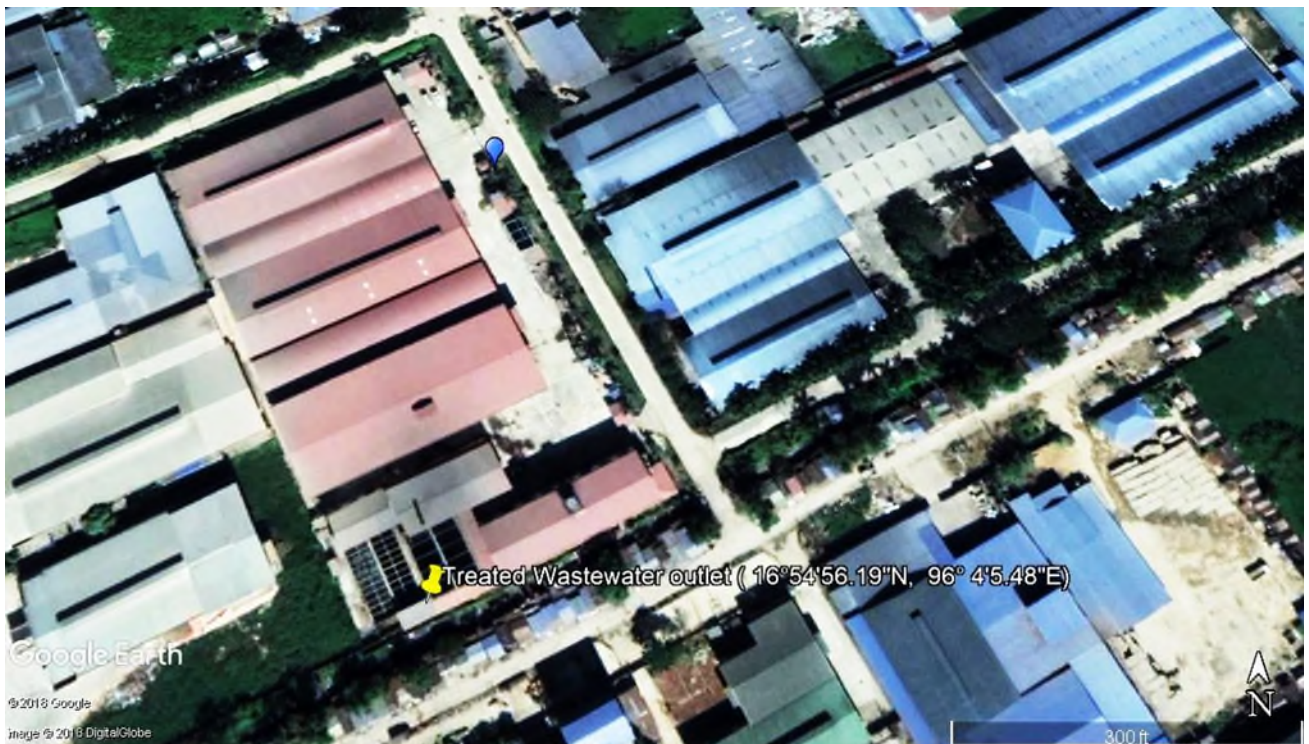
Figure 53: Treated Wastewater outlet ((16°54'56.19"N, 96° 4'5.48"E)
