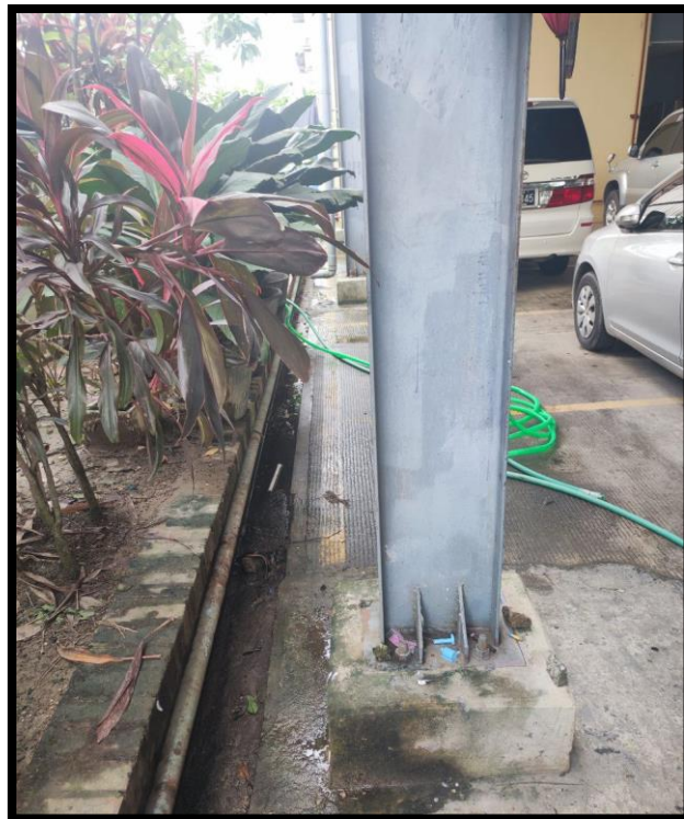
Figure 3-17 Photos of Drainage System
