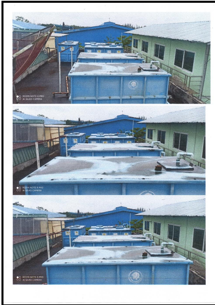
Figure 3-14 Photos of Water Supply
