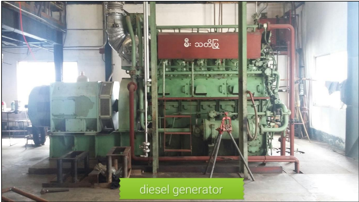
Figure 3.6: Diesel Generator
