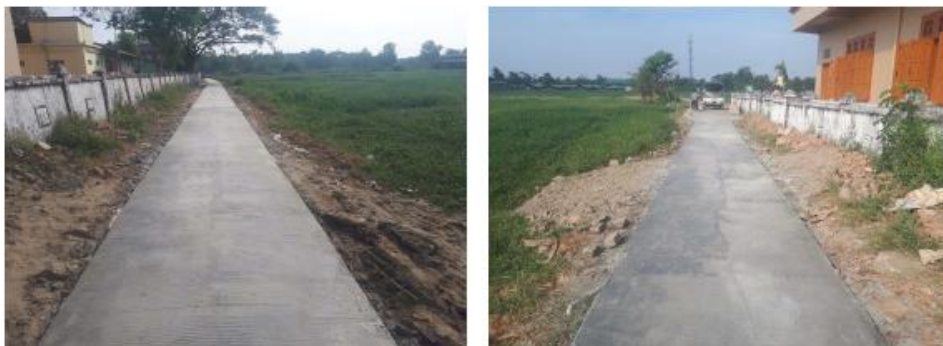
Figure 8-4 Crossroad to bridge
