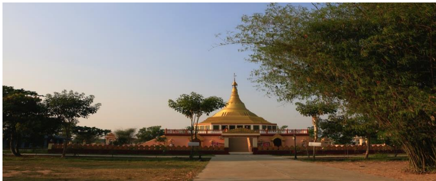
Figure 4-83 Photo of North Iccapunna Stupa
