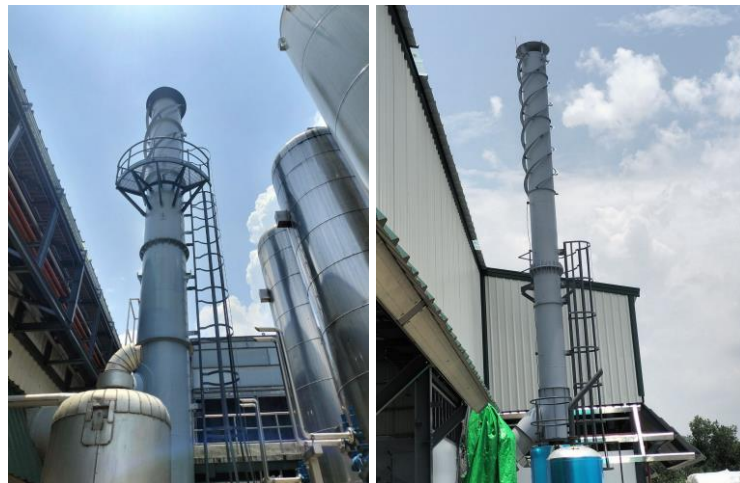
Figure 3-14 photos of boiler chimney-stack
