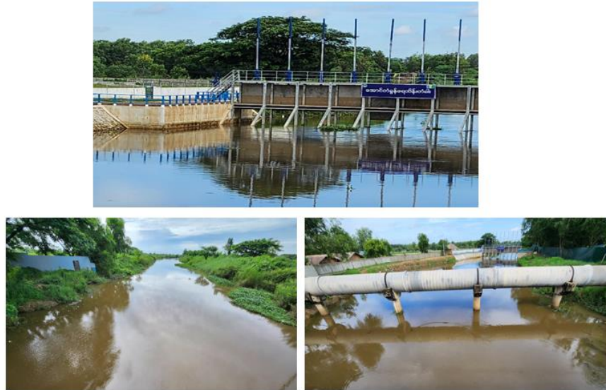
Figure 4-57 visual condition of Barlar creek August 2023
