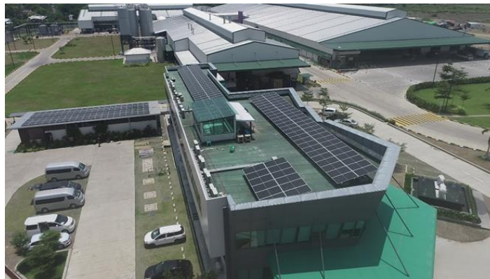
Figure 3-63 photo of solar energy panel on roof of buildings
