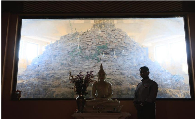
Figure 4-85 Photo of Interior view of Iccapunna Stupa in original brick structure preserved by encasing with new RC structure
