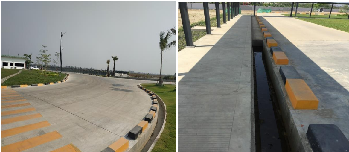
Figure 3-26 Storm Water and Drainage System
