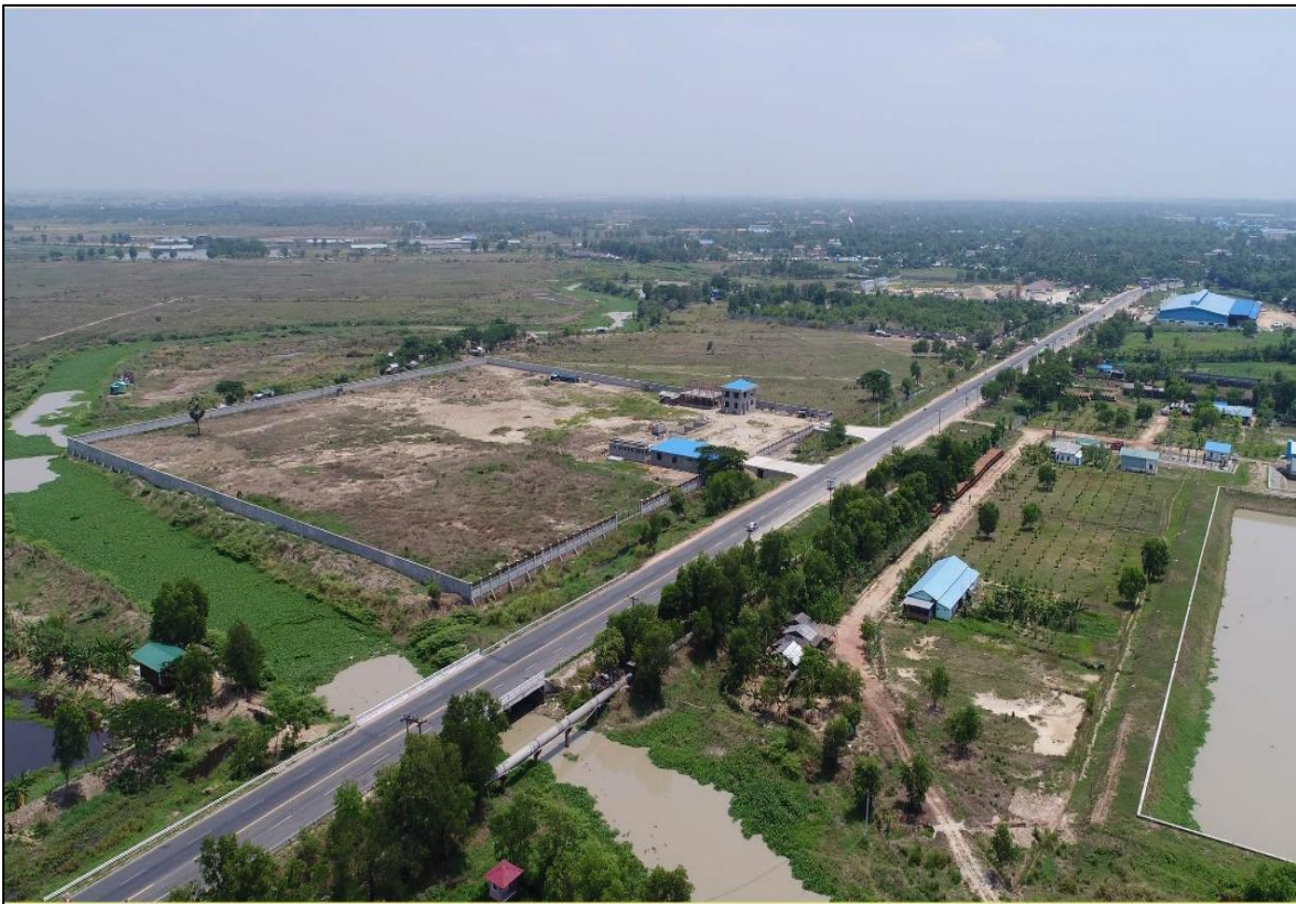
Figure 4-9 North-West View of the Project Site
