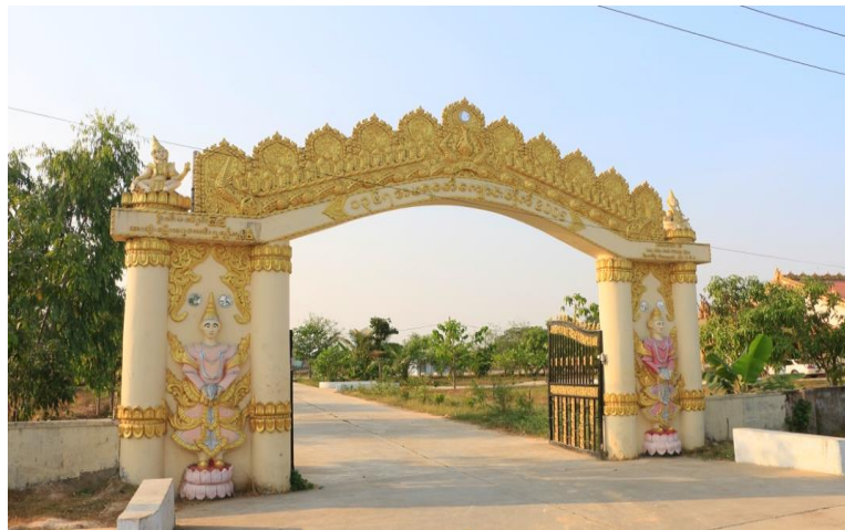
Figure 4-84 Photo of The Façade of Amaravati Monastery Complex (Thai Kyaung Monastery)
