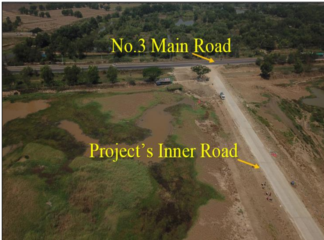
Figure 3-3 On-Site Existing Roads Condition
