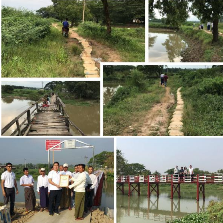
Figure 8-3 Bridge for Ta Kon Taing Village
