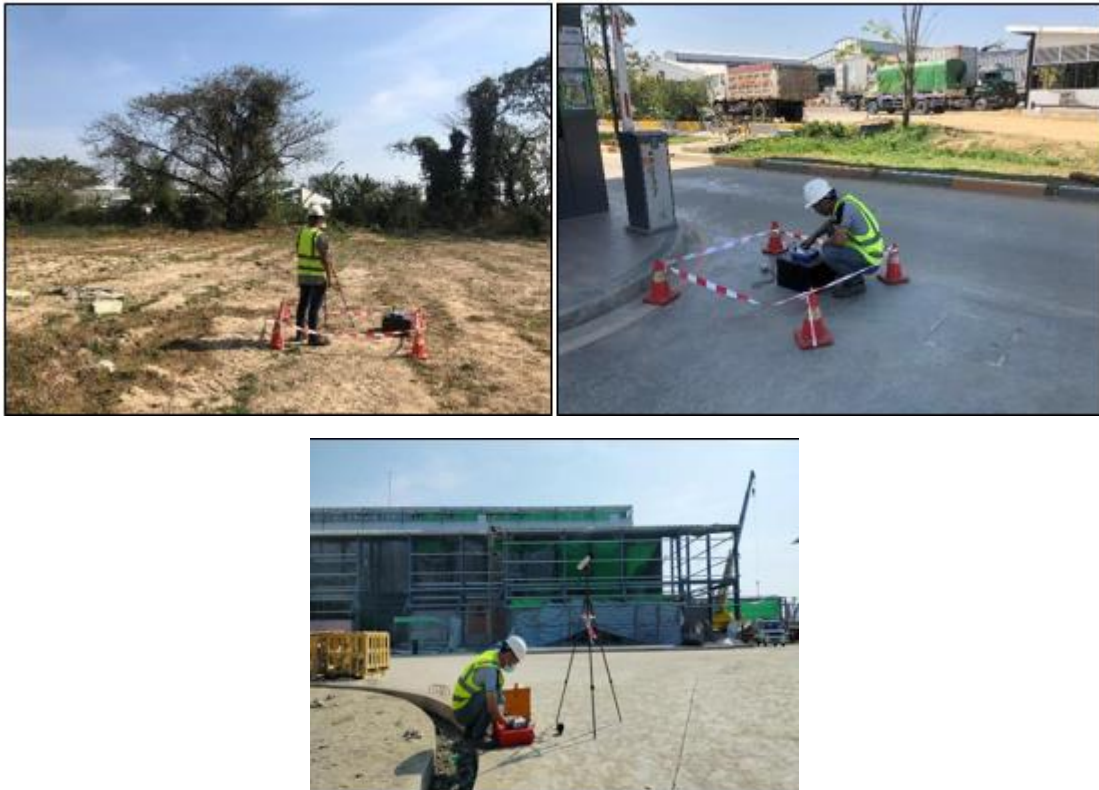
Figure 4-67 photos of vibration measurement
