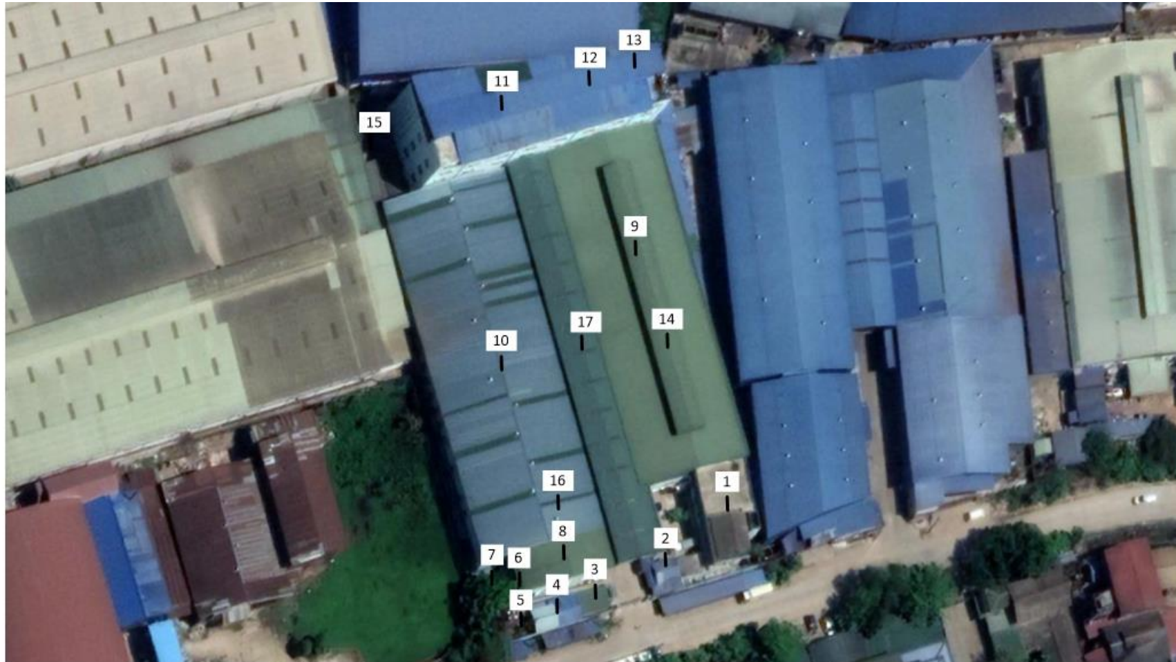
1.Dormitory 2.Security gate 3.Firefighting water tank 4.Generator room 5.Tranformer 6.Diesel Storage area 7.Water Purification System 8.Warehouse 9.Cutting area 10.Sewing area 11.Quality Control 12.Ironing area 13.Boiler room 14.Packing and Final prouduct storage area 15.Toilet 16.Office 17.Canteen
