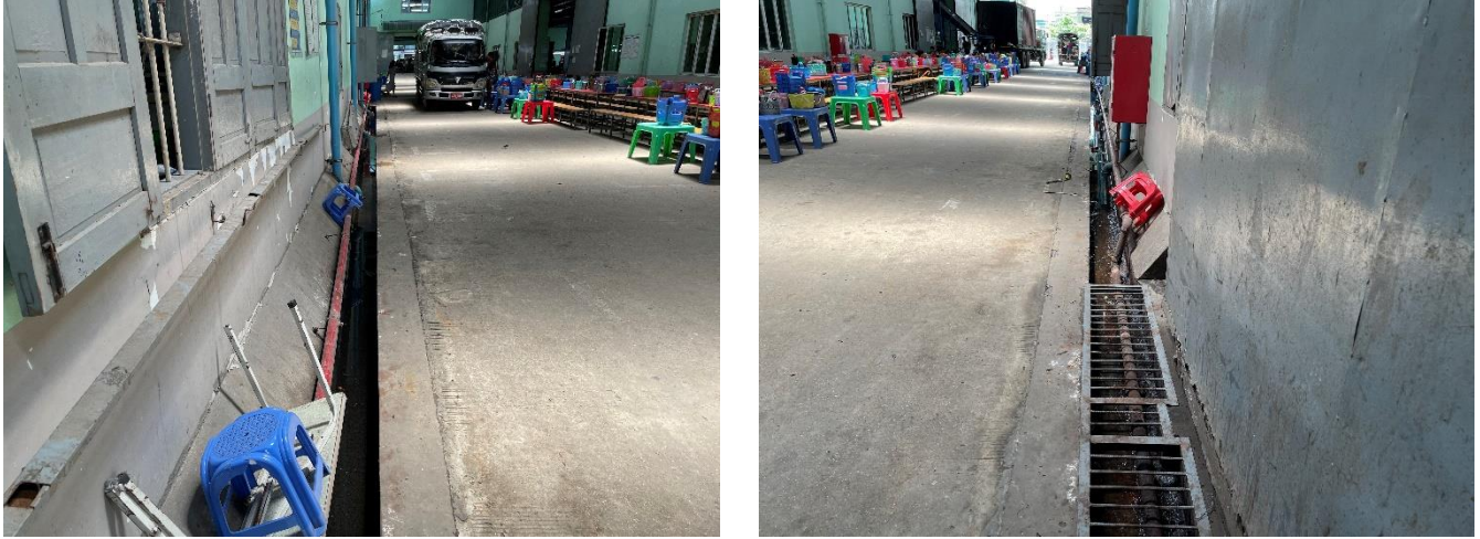
Figure 3-14 Drainage System of Factory
