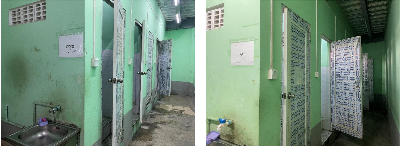
Figure 3-17 Toilet Facilities Photos
