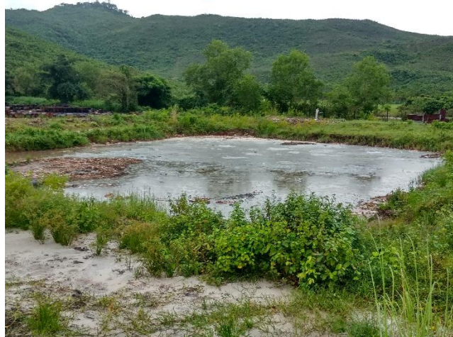
Figure 3.40 First Water treatment pond
