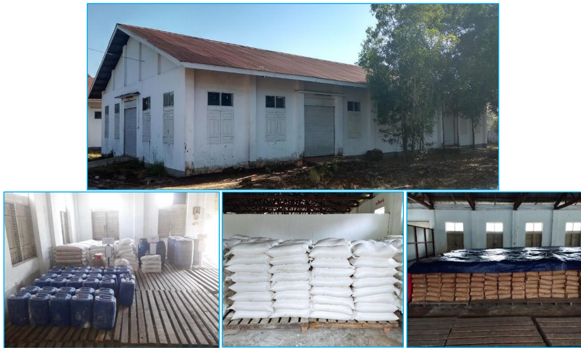
Figure 3.9 Photos of Raw material Storage Building and Storage Conditions
