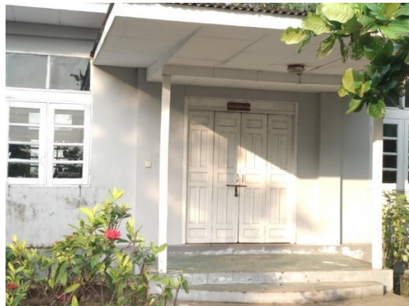
Figure 3.27 Quality Control Office
