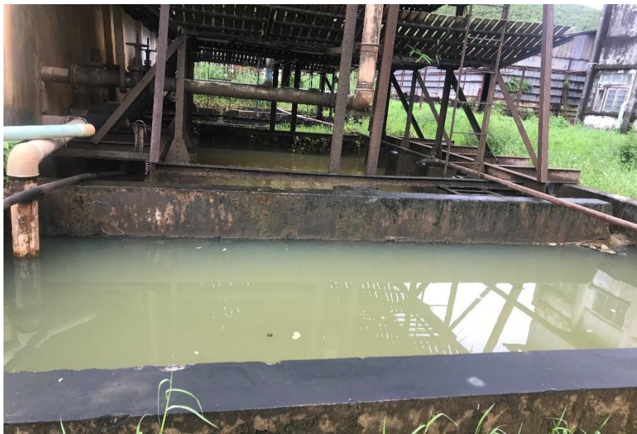
Figure 3.39 Filtration ponds
