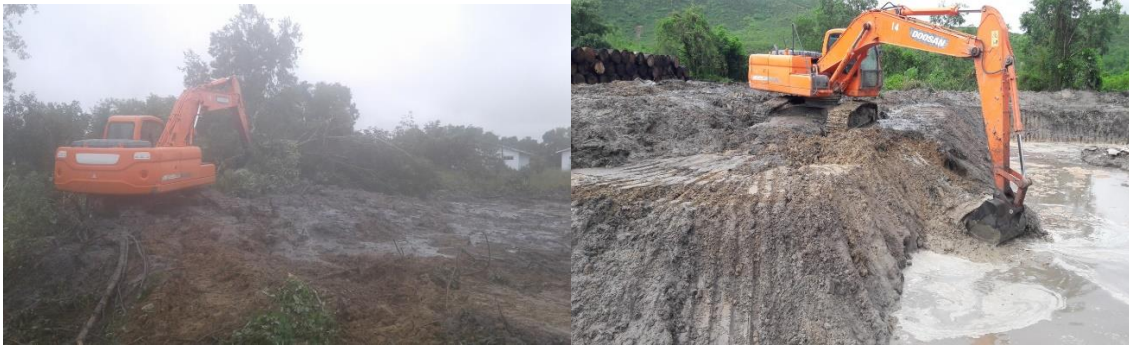
Figure 5.23 Renovations of Waste Water Treatment Ponds
