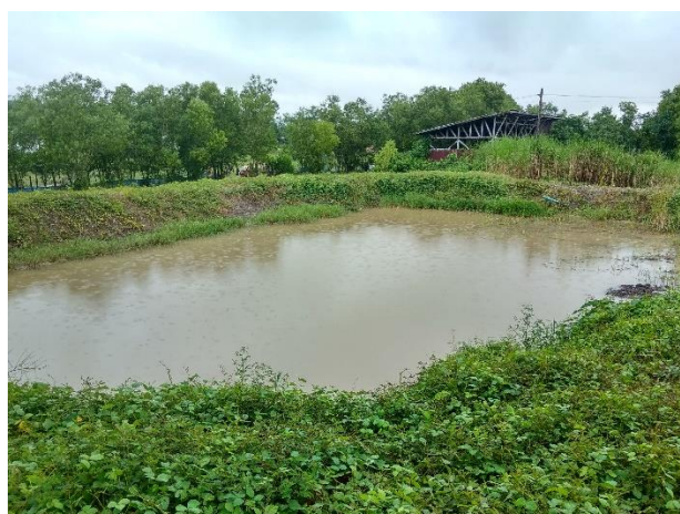
Figure 3.43 Final Water treatment pond
