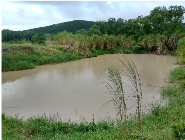
Figure 3.42 Third Water treatment pond
