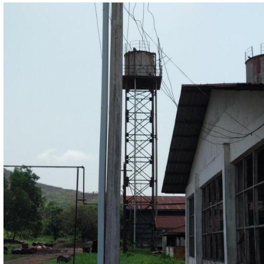
Figure 3.35 Outdoor Over Head Tanks
