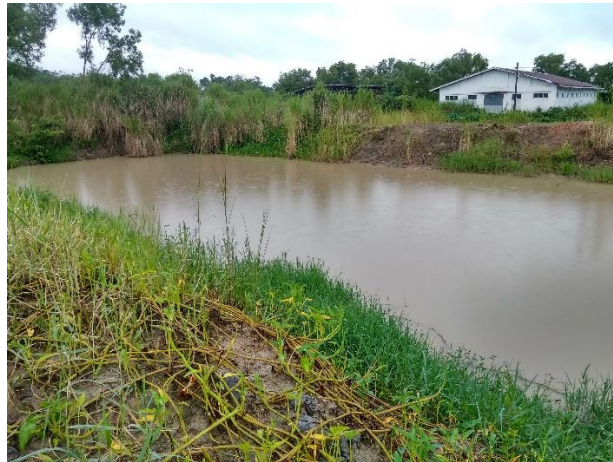
Figure 3.41 Second Water treatment pond
