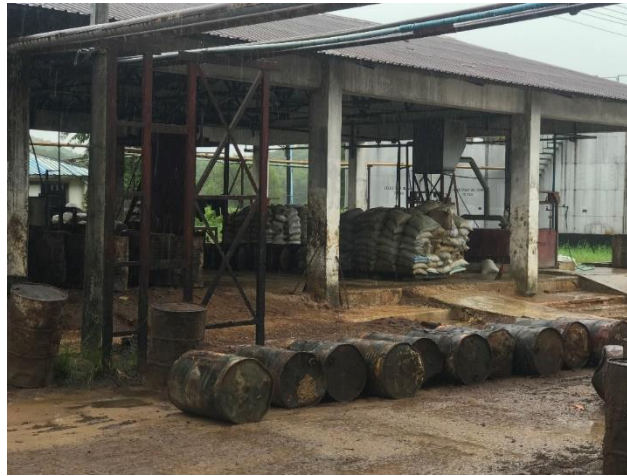
Figure 3.20 Raw Materials Storage Area
