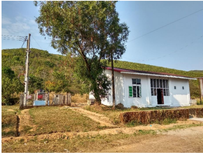
Figure 3.34 Sub Station and Generator Room
