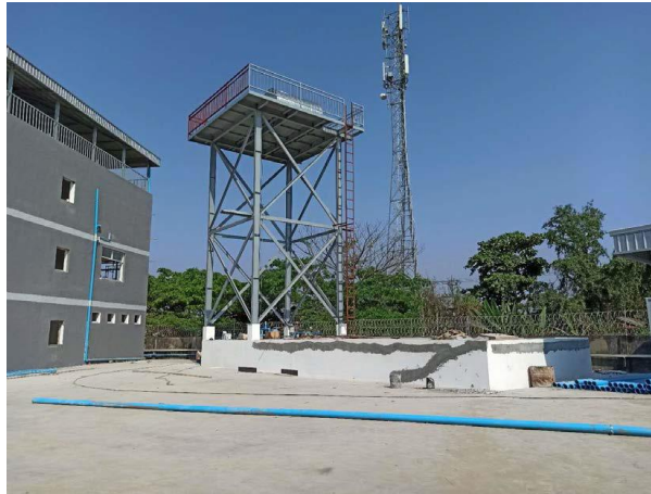
Figure 15. Water Collection from Tube Well Water Concret pool (Concret pool) and upper steel tank
