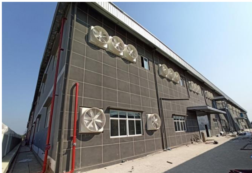
Figure 23. Exhaust Fan are Installed for Ventilation
