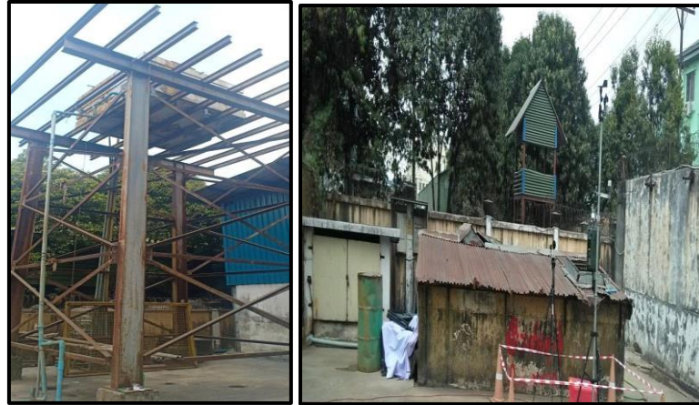
Figure 3-14 Water Storage Tanks for Domestic Usage and Firefighting
