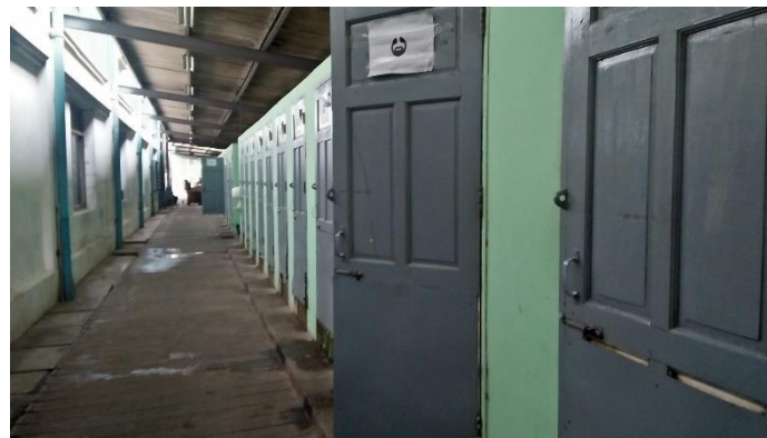
Figure 3-34 Photos of Toilets
