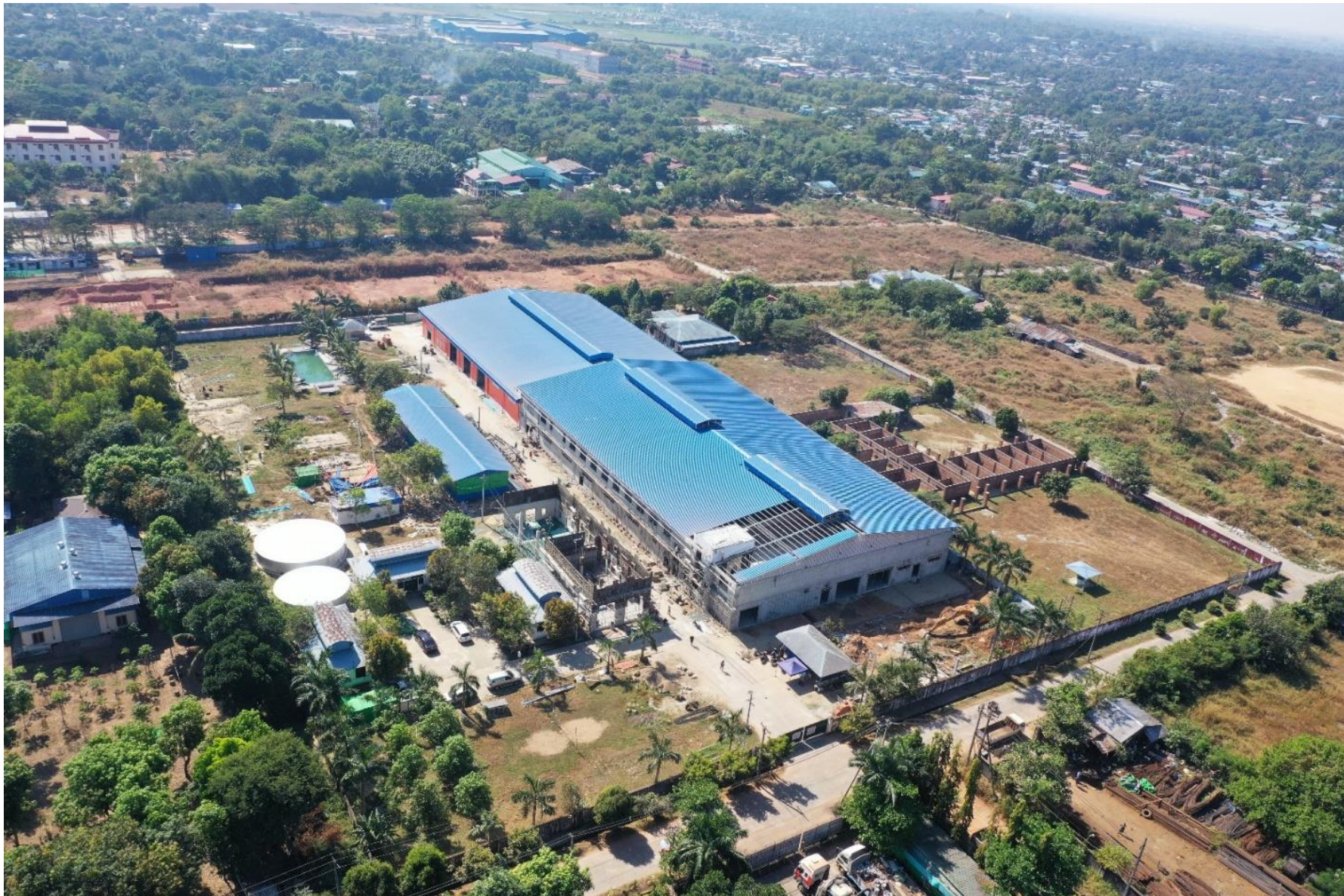
Figure 3-9 Aerial of Proposed Project (December 2020)
