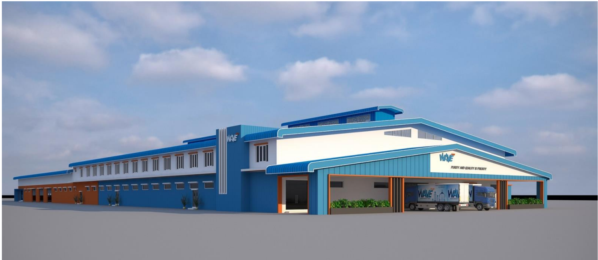
Figure 3-3 Front View of Factory Building
