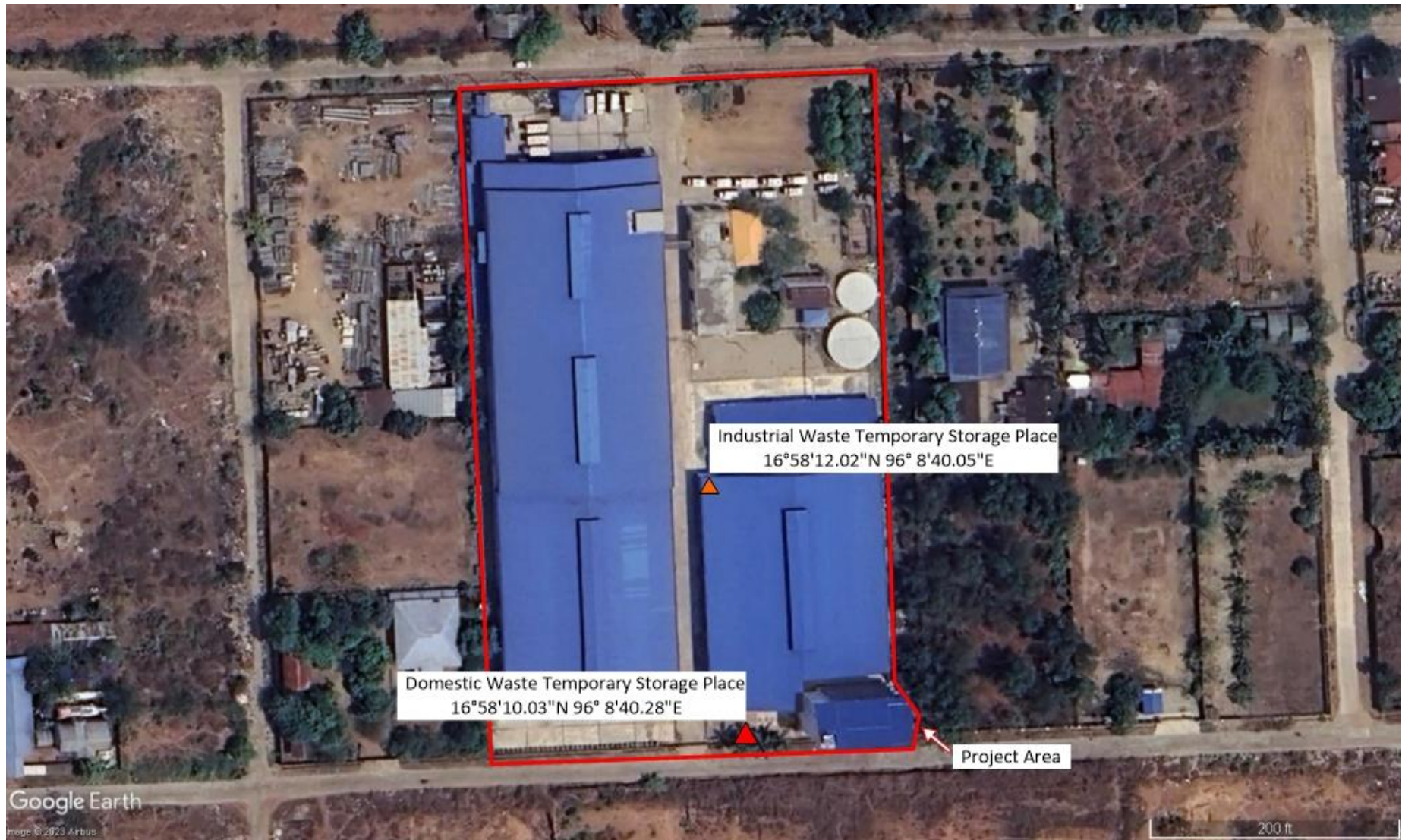
Figure 6-9 Waste Storage Area
