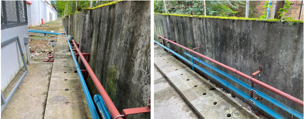
Figure 3-22 Drainage System Photos
