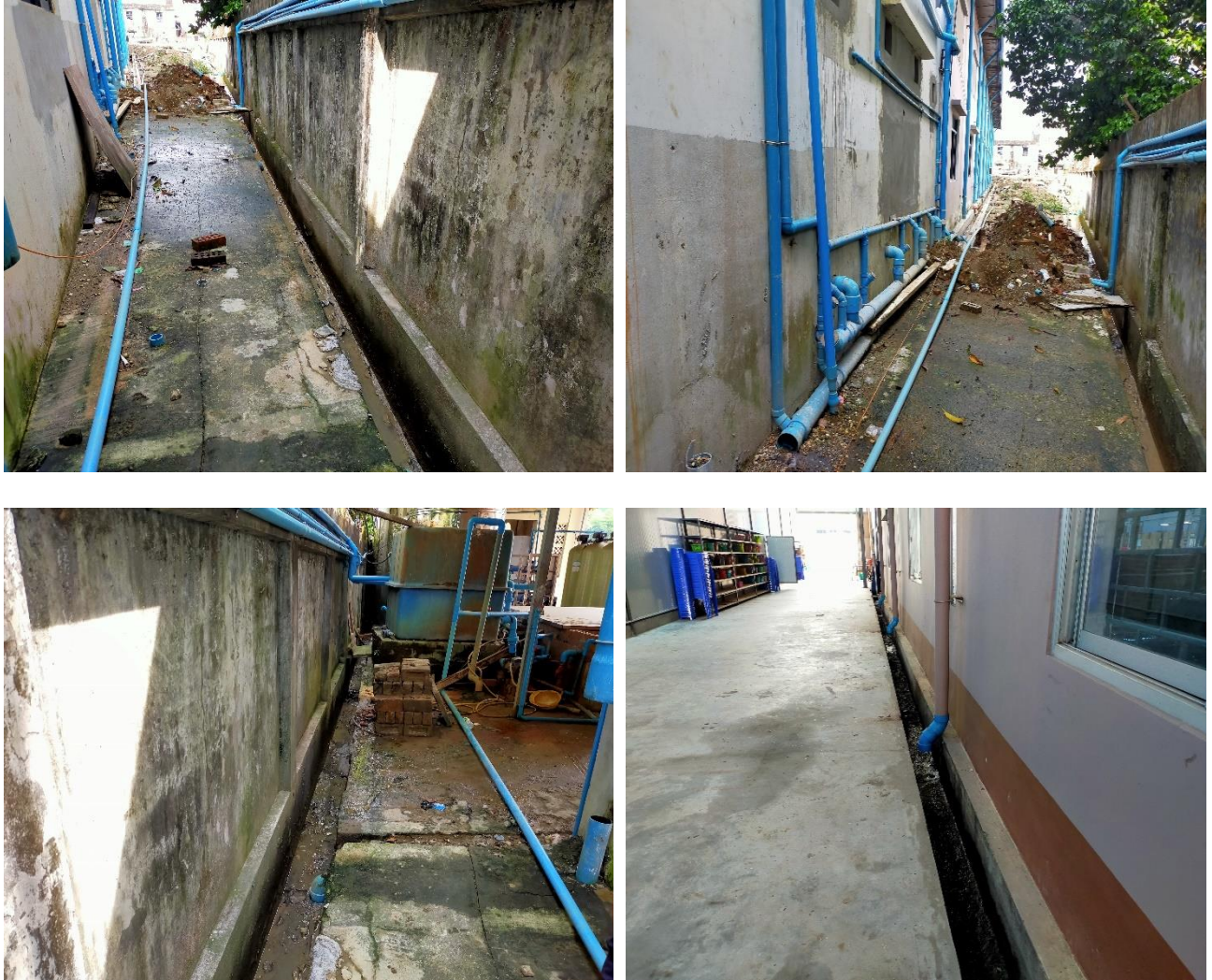
Figure 3-11 Drainage and Toilet facility
