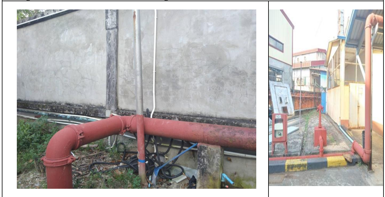
Figure 9.7: Installation of Fire Safety Pipeline
