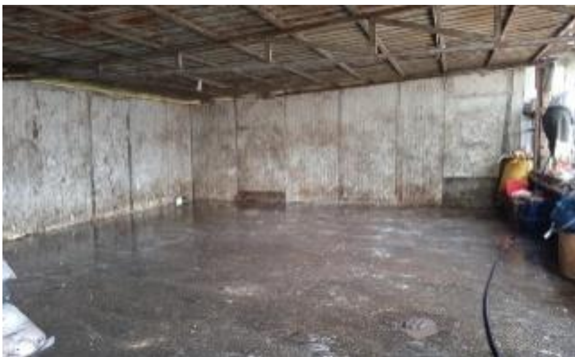
Figure 4.36: Temporary Garbage Tank
