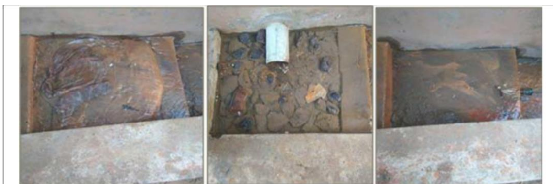
Figure 8.19: Sand and Gravel Filtration of the Premier Factory
