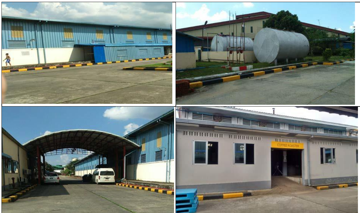
Figure 5.24 Current situation of Lluvia premise (90% of land is concrete)
