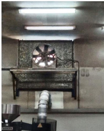
Figure 5.20 : Exhaust Fans in the production rooms
