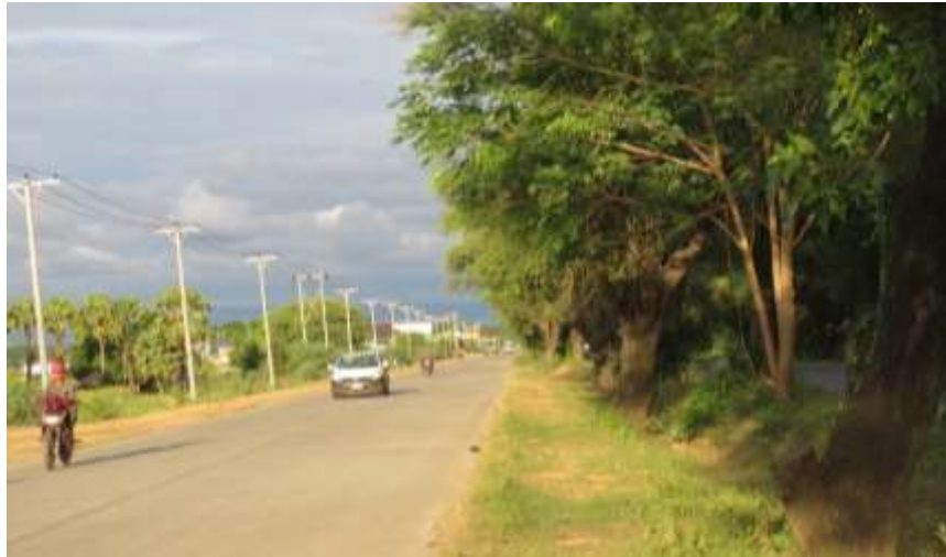
Figure-36: Sagaing-Myitnge road (project site is on the left)
