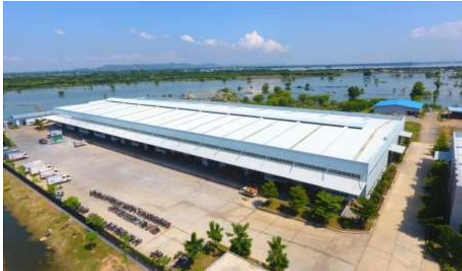
Figure – 8: Raw Material Warehouse
