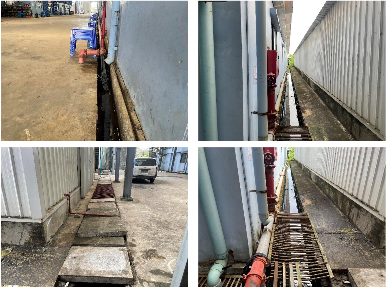
Figure 3-12 Drainage System of Factory
