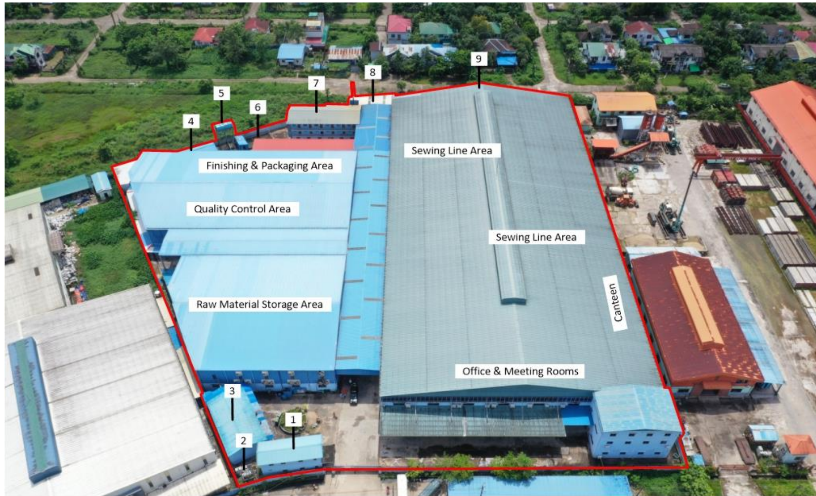
1. Security Gate 2. Transformer 3. Generator Room 4. Fabric Scrap Storage Area 5. Overhead Tank 6. Water storage tank 7. Dormitory 8. Boiler Room 9. Toilets
