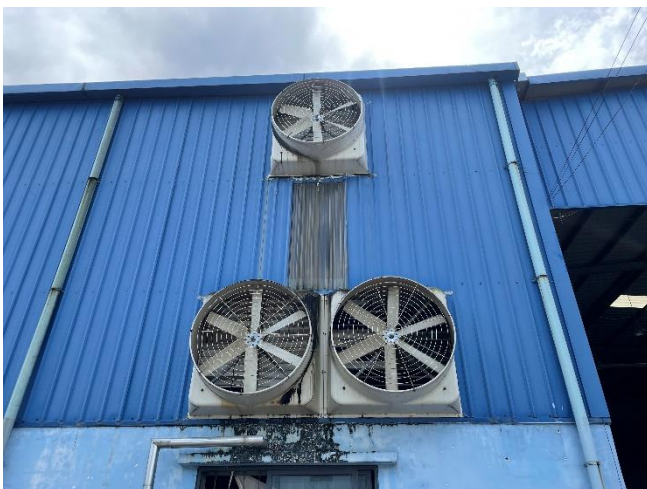
Figure 3-14 Ventilation System
