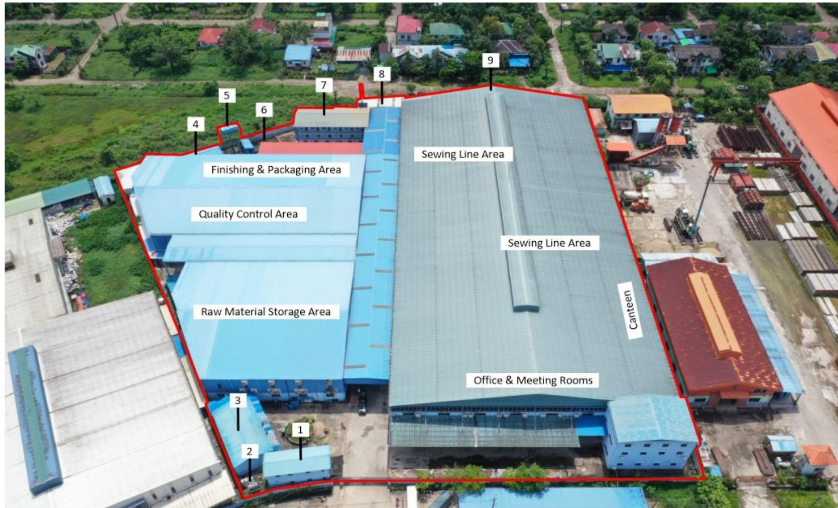
1. Security Gate 2. Transformer 3. Generator Room 4. Fabric Scrap Storage Area 5. Overhead Tank 6. Water storage tank 7. Dormitory 8. Boiler Room 9. Toilets
