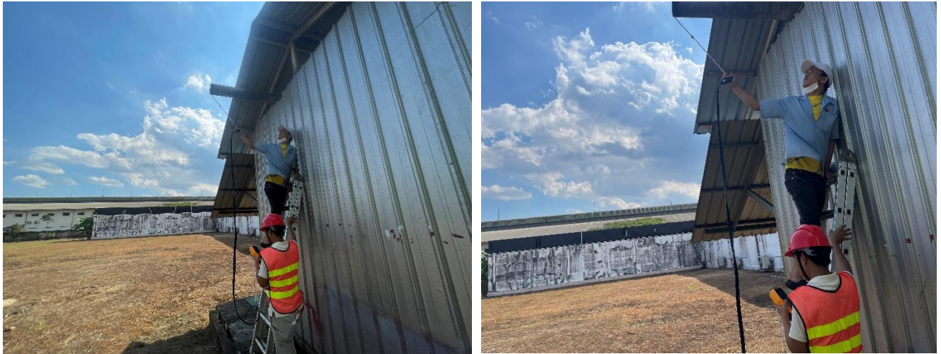
Figure 4-2 Stack Emission of the generator
