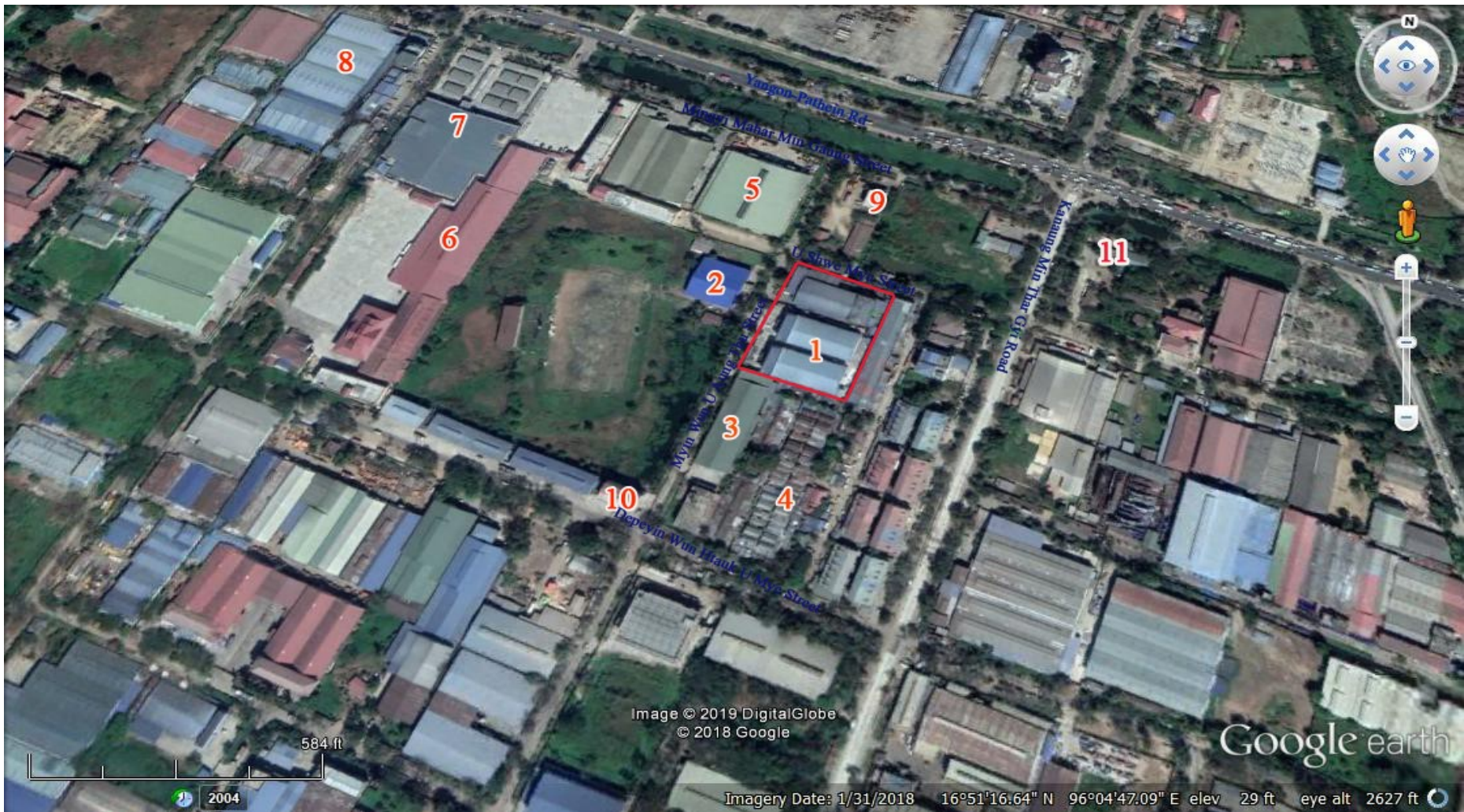
Figure – 37: Satellite image of project site and other facilities in its environs
