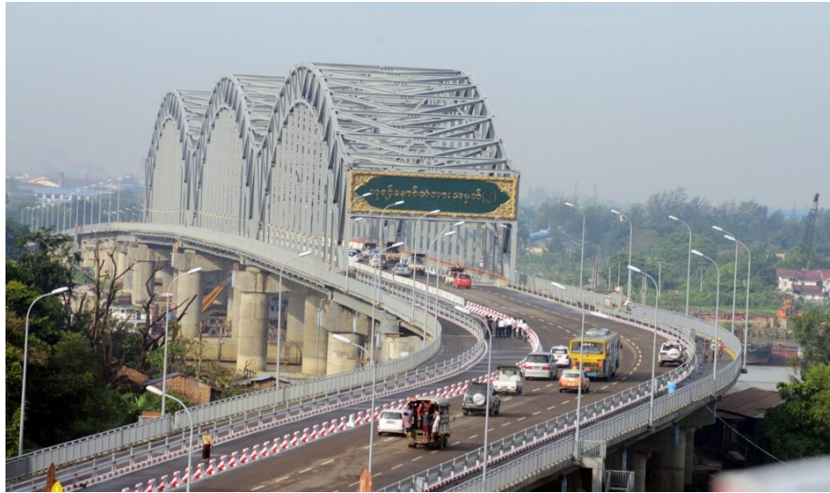
Figure-48: Bayint Naung Bridge
