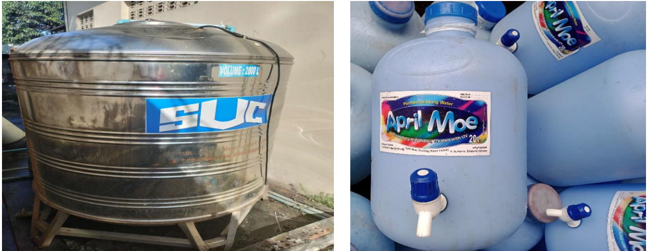
Figure 3-11 Water storage tank and drinking water supply
