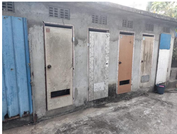
Figure 3-15 Toilet Facility Photo
