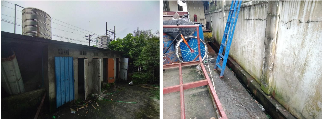
Figure 5-4 Drainage and Septic tank in project area
