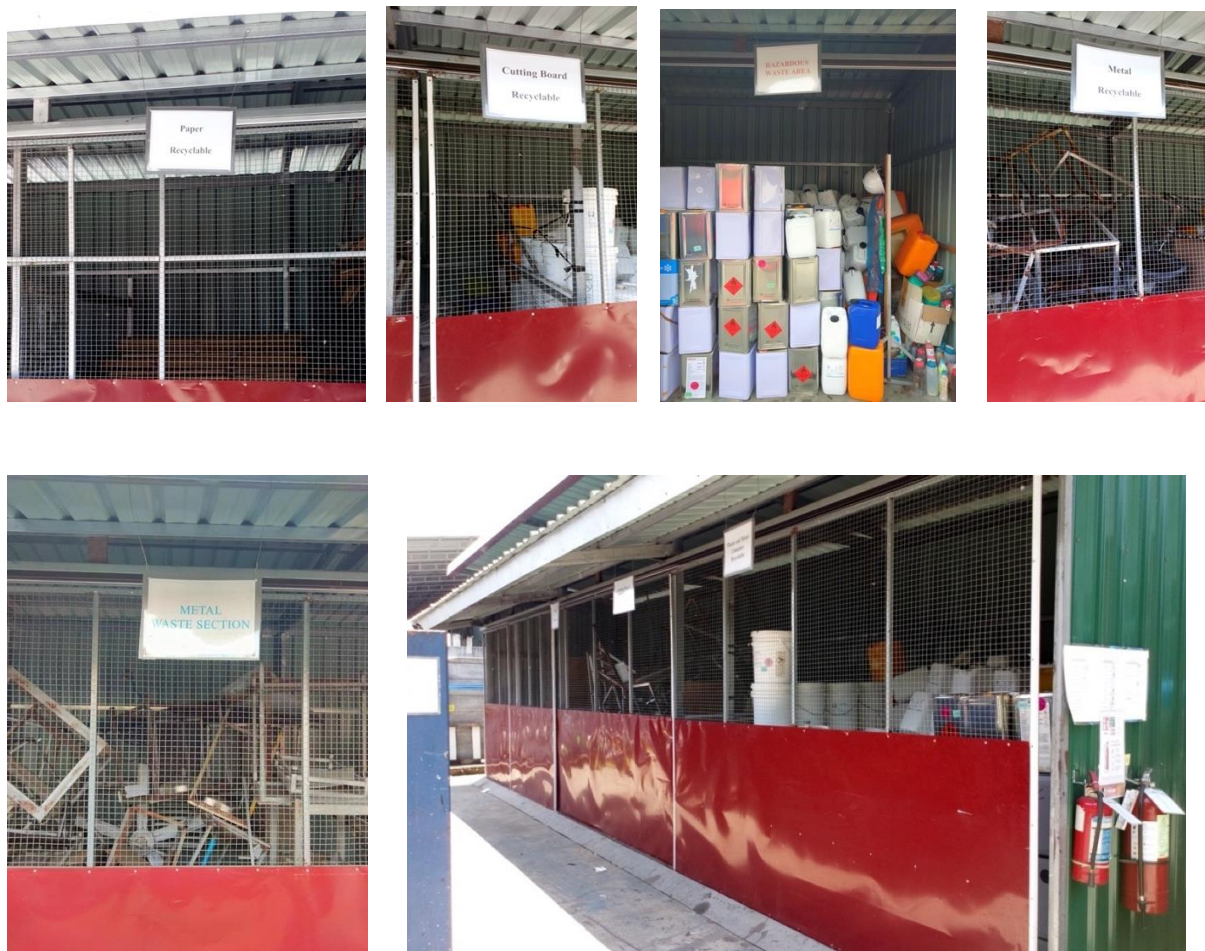
Figure 3.44 Temporary Solid Waste Storage Area
