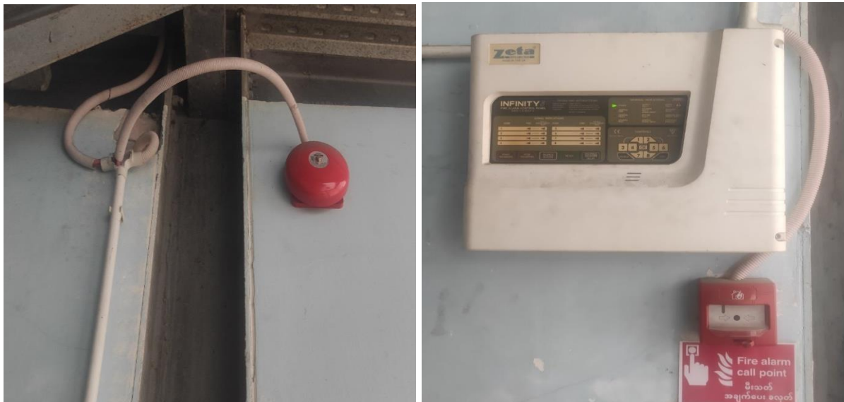
Figure 6.2 Electric Fire Alarm System
