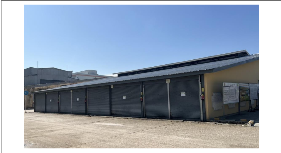
Chemical Storage Room
