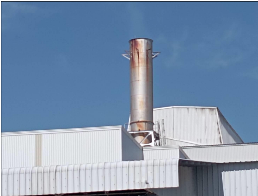
Figure 8-8 Current Condition of Chimney
