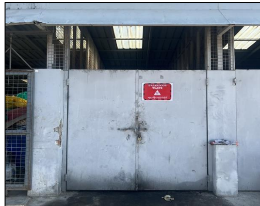
Hazardous Waste Storage Site
