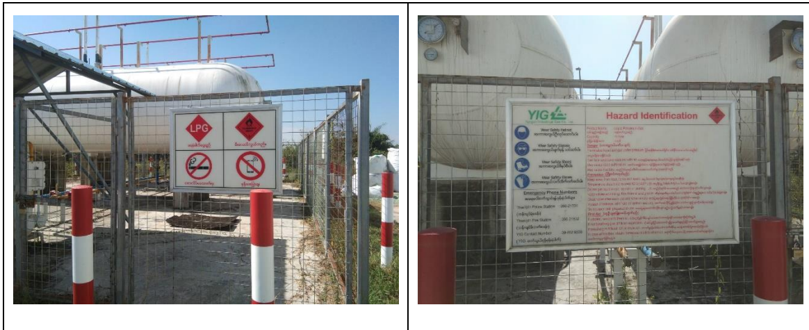
Figure 8-19 The Current Condition of LPG Storage Area
