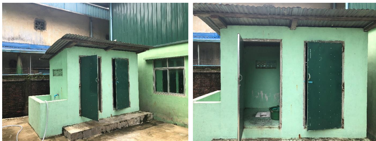
Figure 5-3 Toilet Facilities in factory at Myanmar Green Start Energy Factory
