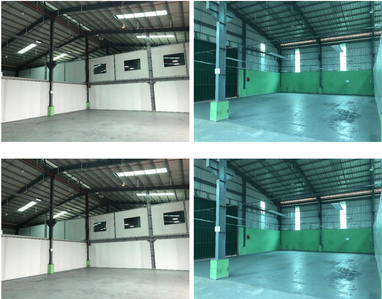
Figure 3-1 Construction Phase of Myanmar Green Start Energy Factory
