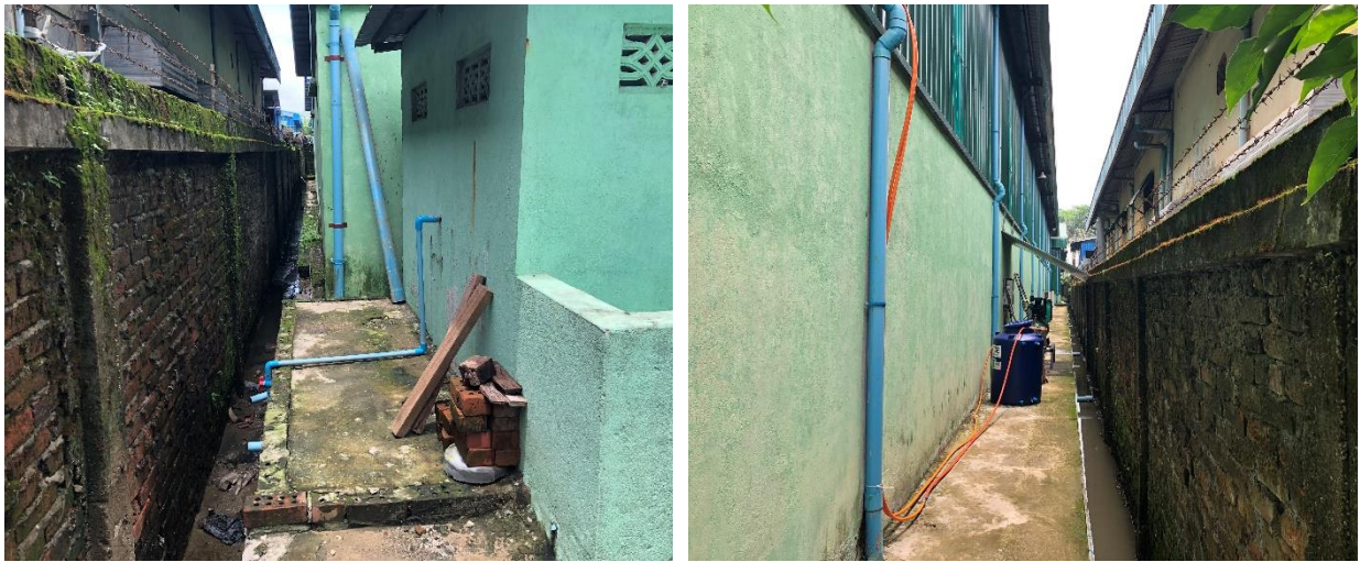
Figure 3-12 Rainwater drainage in factory compound
