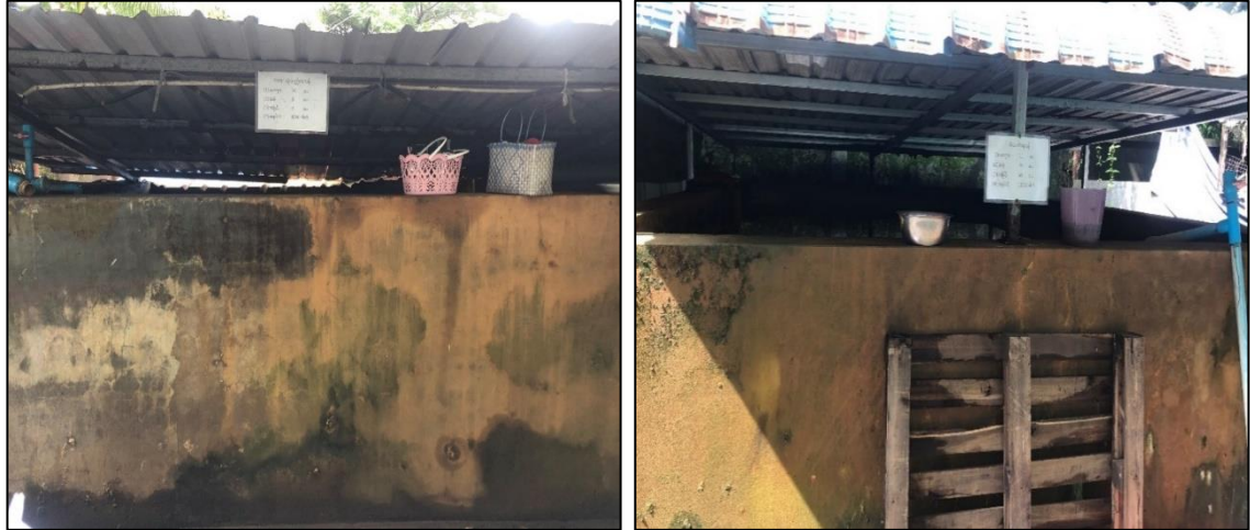
Figure 3-15 Photos of Water Supply
