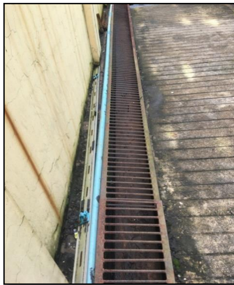
Figure 3-18 Photo of Drainage System
