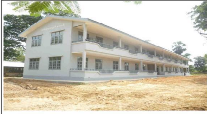
B.E.H.S (Myo Hla) (Two-Storey Building) Donated Amounts : The whole building Donated Year : 13.11.2015 Address : Yedashe Township, Taungtha District, Bago Region
