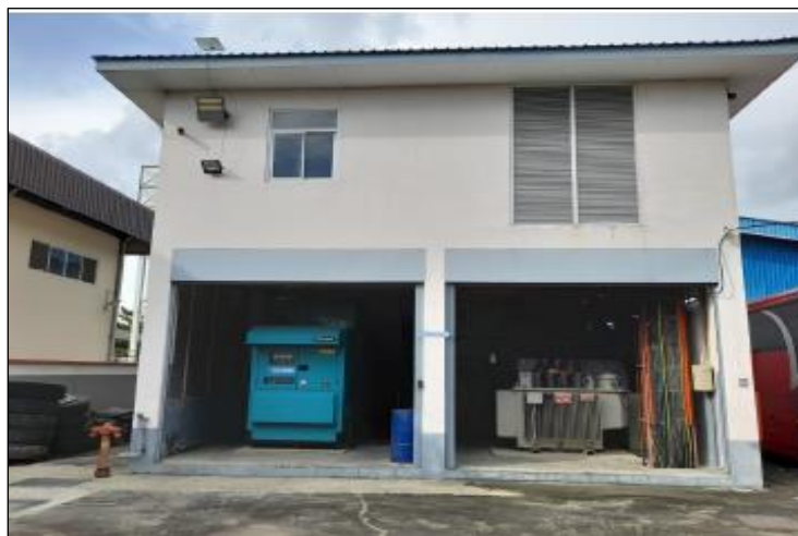
Figure 3.18 Power Station Building
