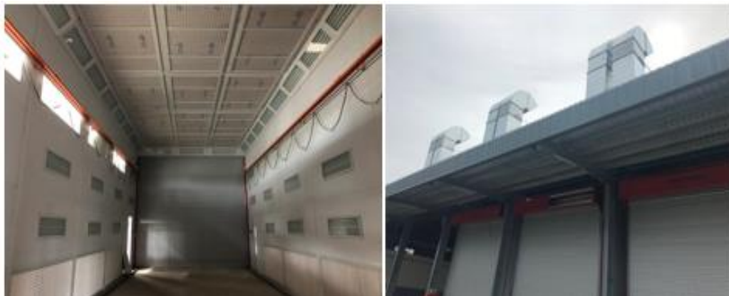
Figure 5.5 Activated carbon Filter
