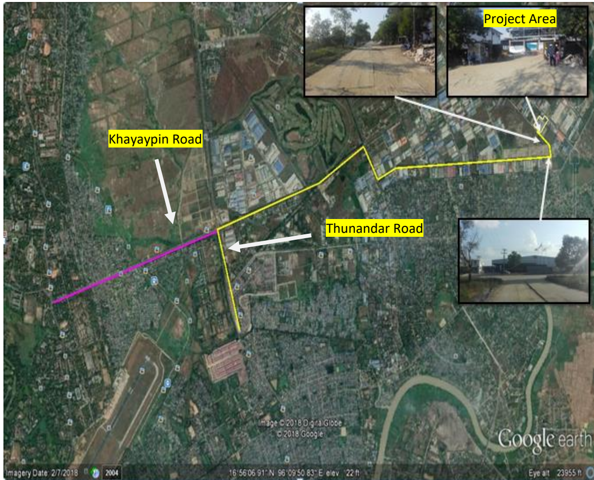
Figure 3.2 Assess Road around the Project Area
