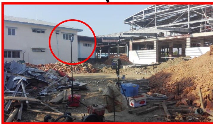
Figure 4.12 Locations of Ambient Noise Measuring Point
