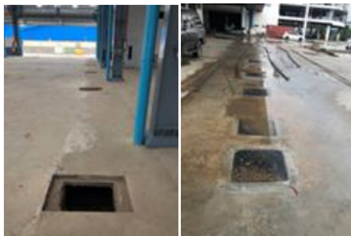
Figure 3.30 Photos of concrete pavement and Drain Channel
