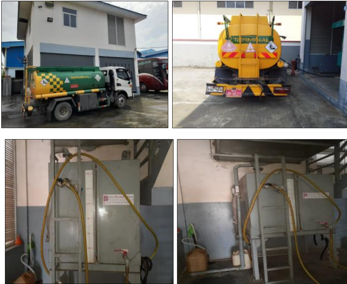
Figure 3.19 Photos of Diesel Transportation and Storage Tank
