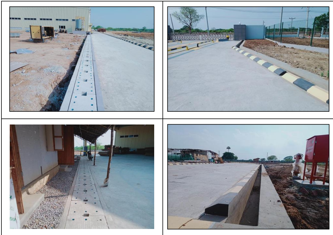
Figure 3-23 Current Condition of Drainage Channel of the Proposed Factory
