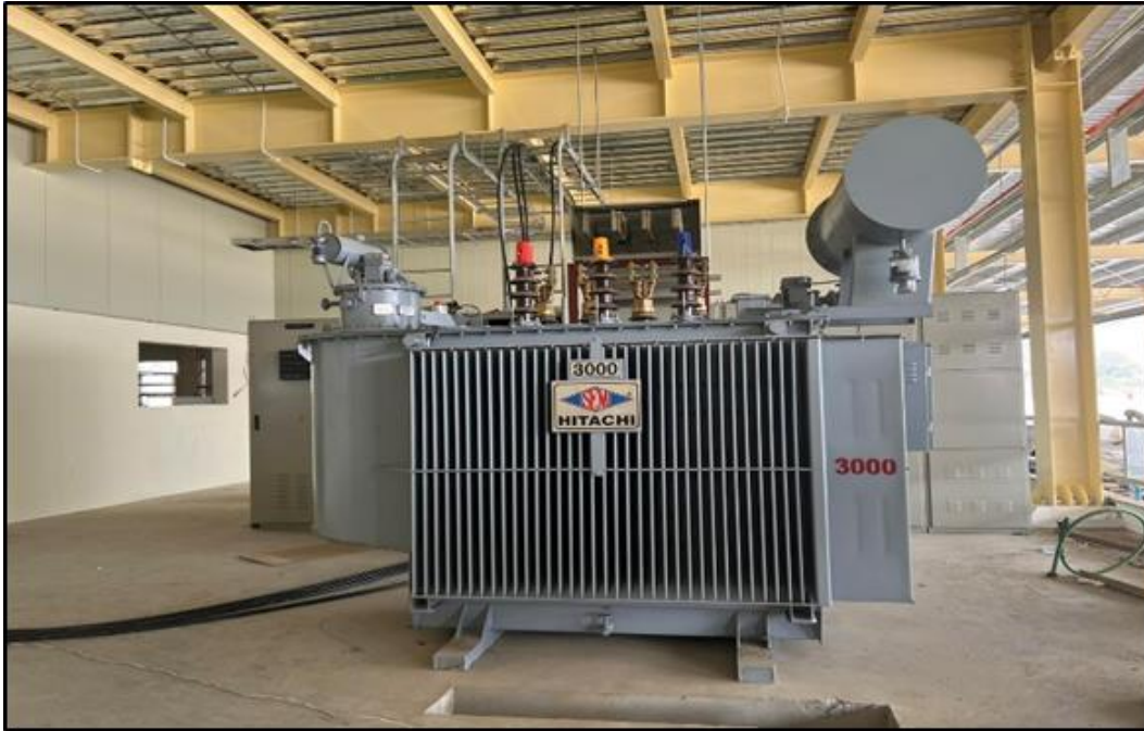
Figure 3-24 3,000 KVA Transformer
