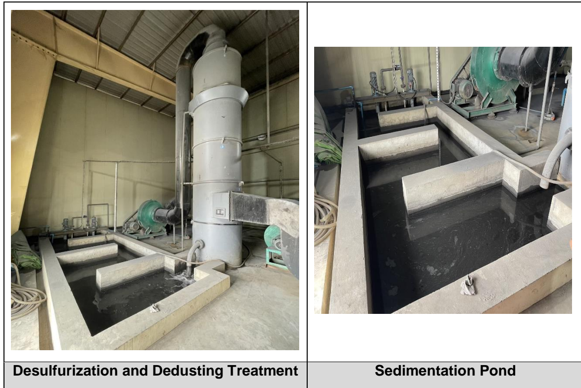
Figure 3-29 Swirl Water Film Desulfurization Dust Collector
