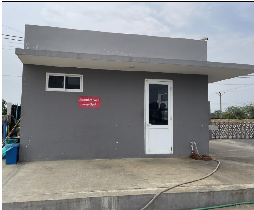
Figure 8-13 Assembly Point of the Proposed Factory
