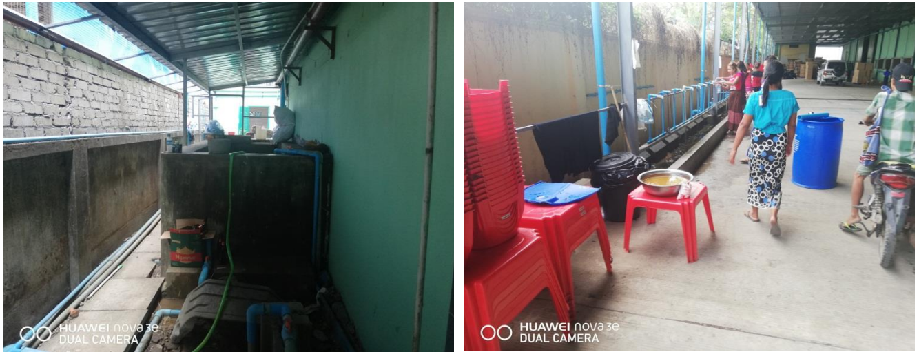
Figure 3-1 Water Storage Tank and Drinking Water Supply
