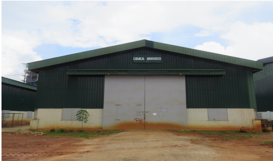
Figure – 27: Chemical Warehouse
