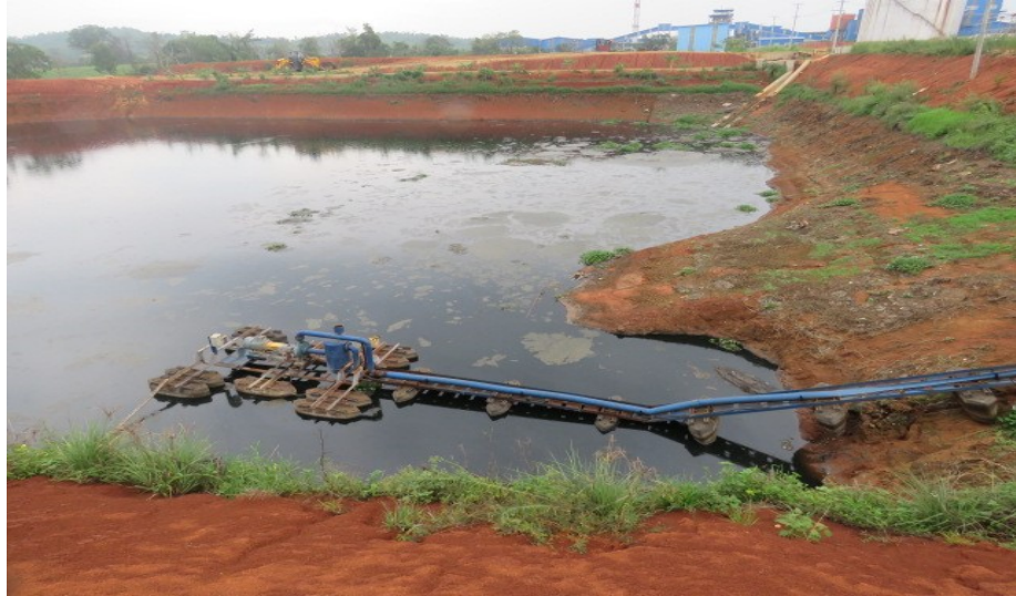
Figure-73: The final waste water pond (part of the water is pumped up and used for watering sugar cane plantation)
