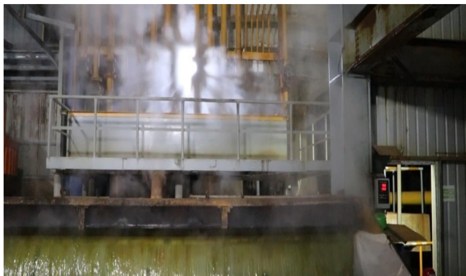
Figure-59: Pouring clear juice from sedimentation tank
