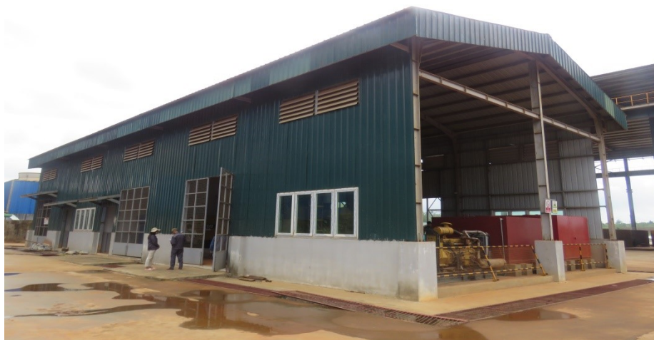
Figure-40: Transformer and generator house
