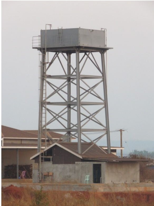
Figure-43: Overhead tank and concrete ground tank (water purification system is inside)
