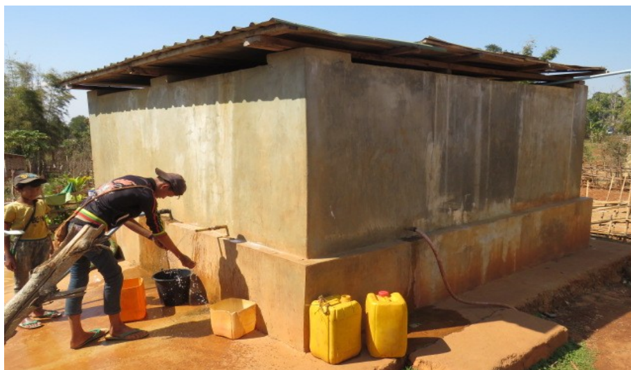
Figure-107: Concrete water pond constructed by the company for Hsen Taw Village
