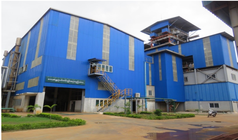
Figure – 22: Turbine house and control room
