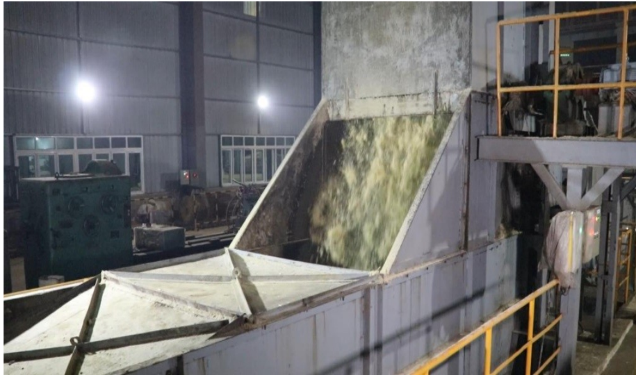
Figure-52: Conveying shredded sugar cane to mill
