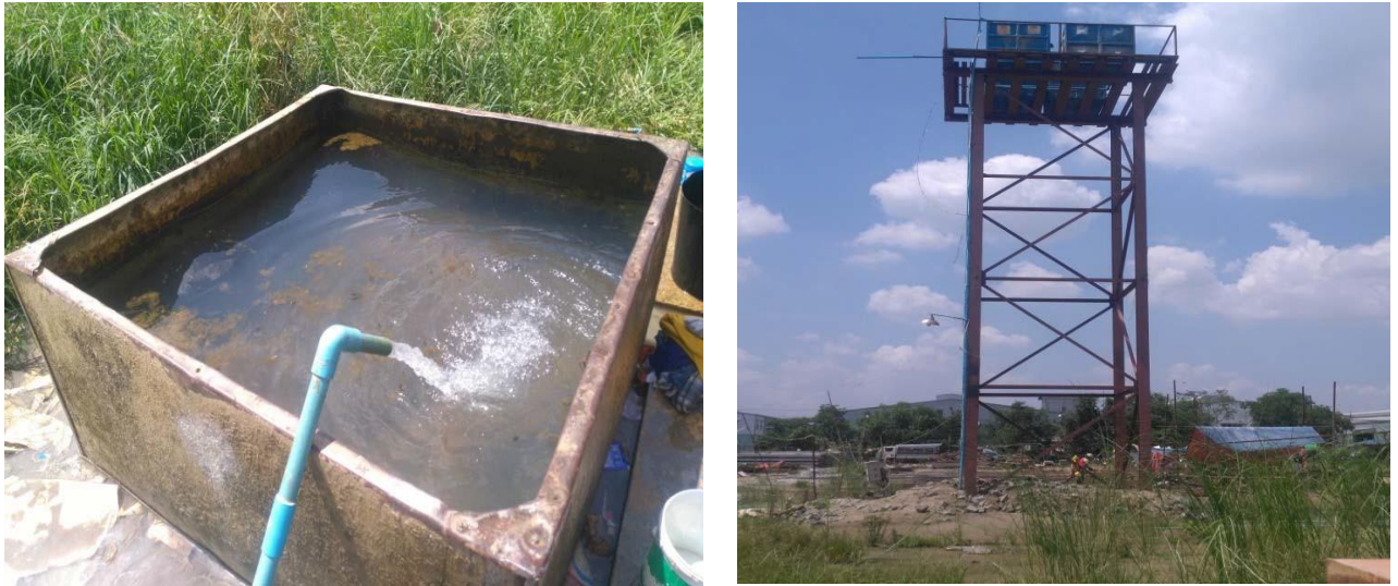
Figure 4.15: Water storage tanks
