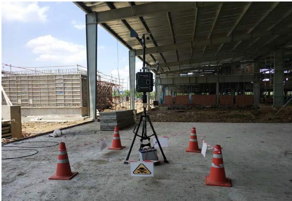
Figure 5.2 Ambient air monitoring at the LPG Tank (Location-1)
