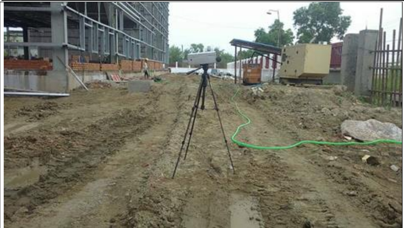
Figure 5.9 Noise monitoring station nearby the project site building
