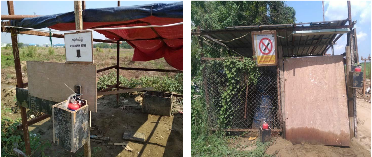
Figure 4.14: (a) Fire extinguishers are installed at the special areas during the construction phase
