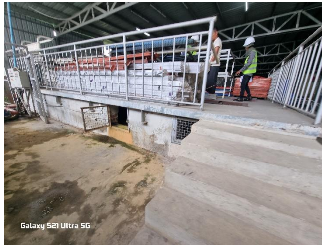
Figure 3-10: Underground water tank for domestic use
