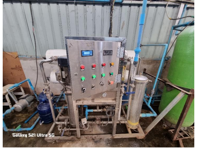
Figure 3-9: R.O System for Drinking Water
