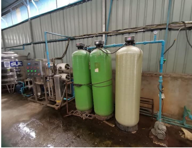
Figure 3-9: R.O System for Drinking Water
