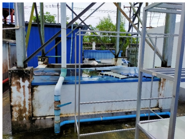
Figure 3-8 Underground water storage tank and water supply
