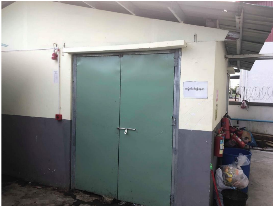
Temporary waste storage room
