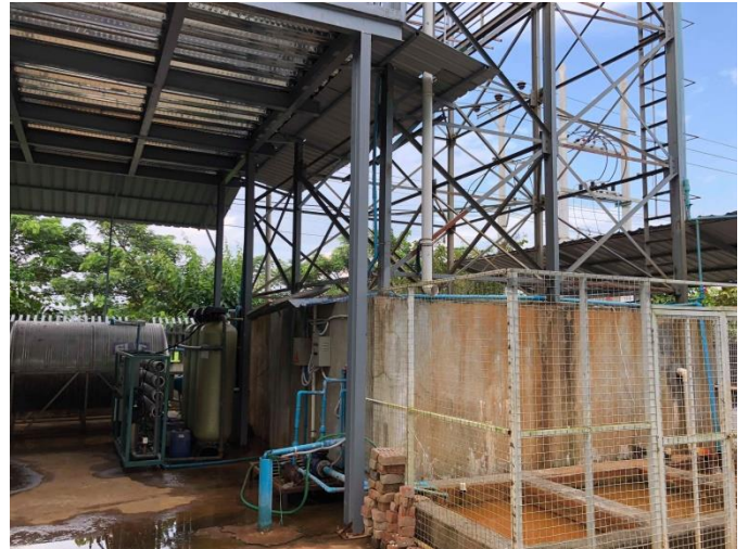
Ground Water Tank
