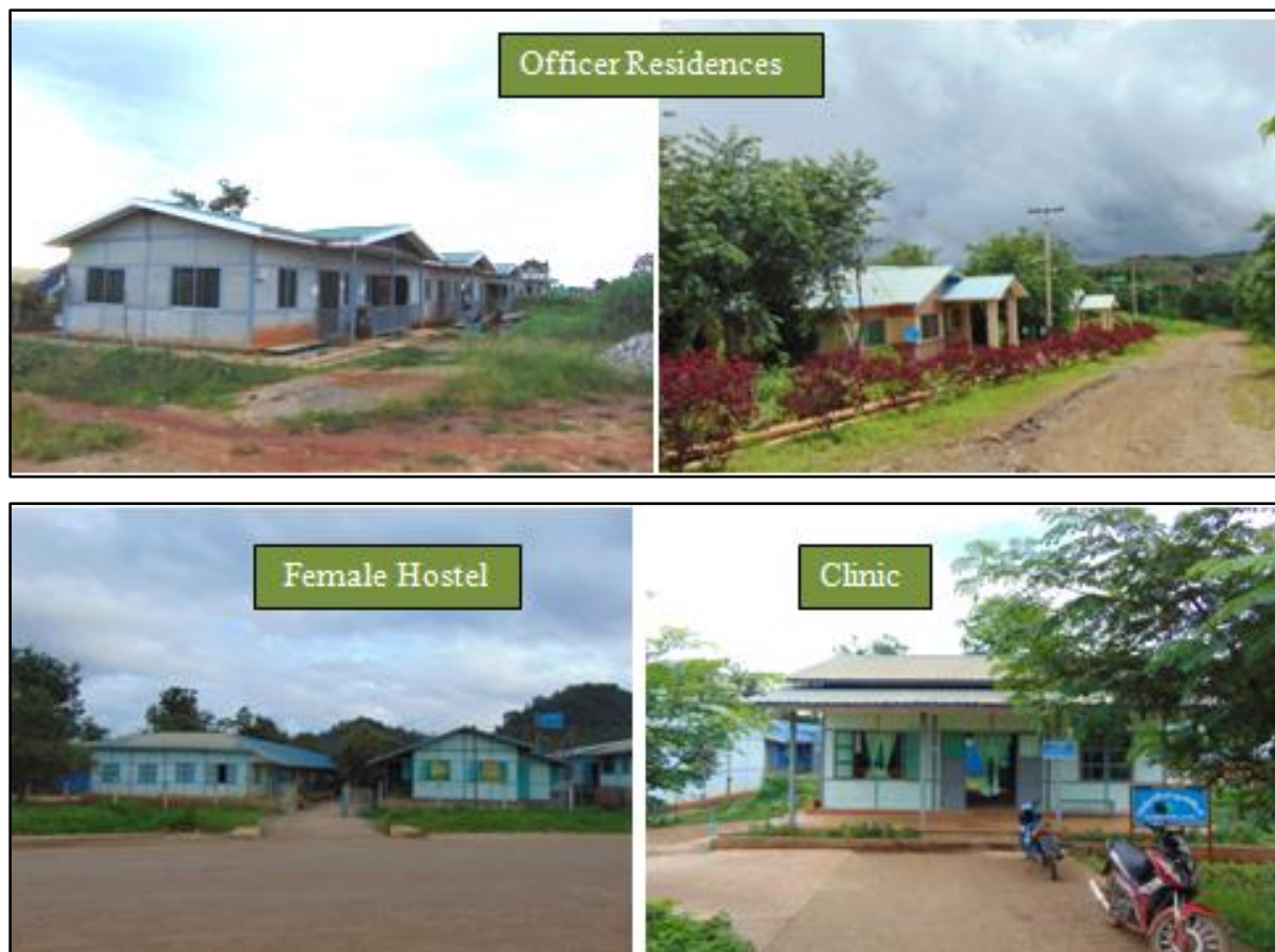
Figure 7-5 Facilities Provided as Social Welfare Program
