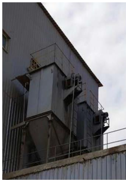
Figure 3-27 Photos of EP Dust Controller and Bag Filters
