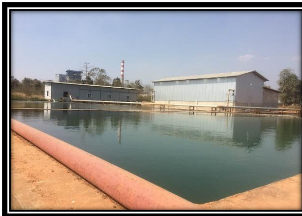
Water tank (15 million gallon)
