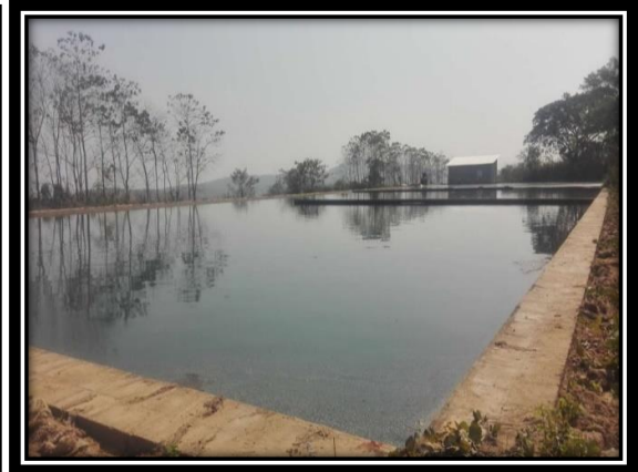
Water tank (21 million gallon)
