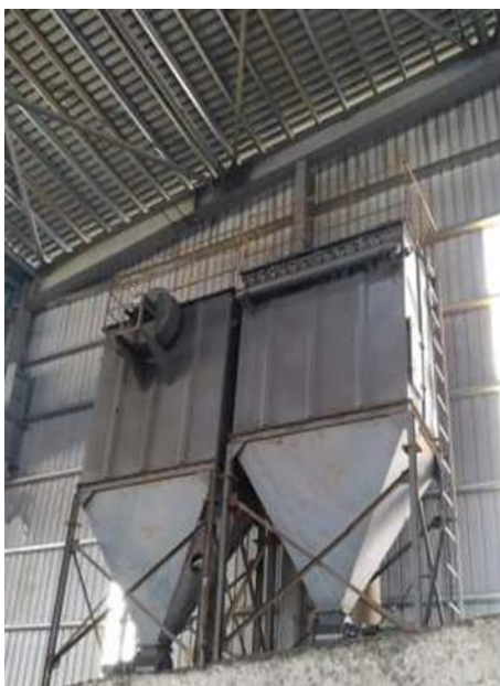
Figure 3-27 Photos of EP Dust Controller and Bag Filters
