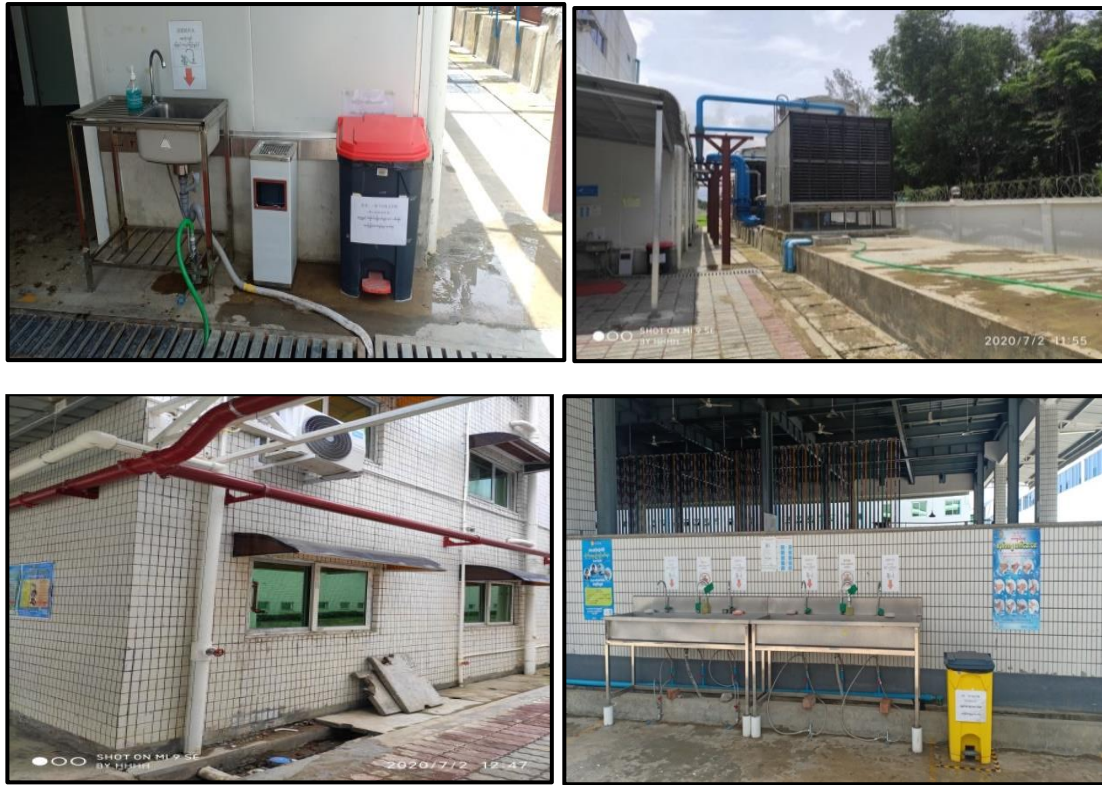
Figure 3-16 Basins and Drains in the Factory
