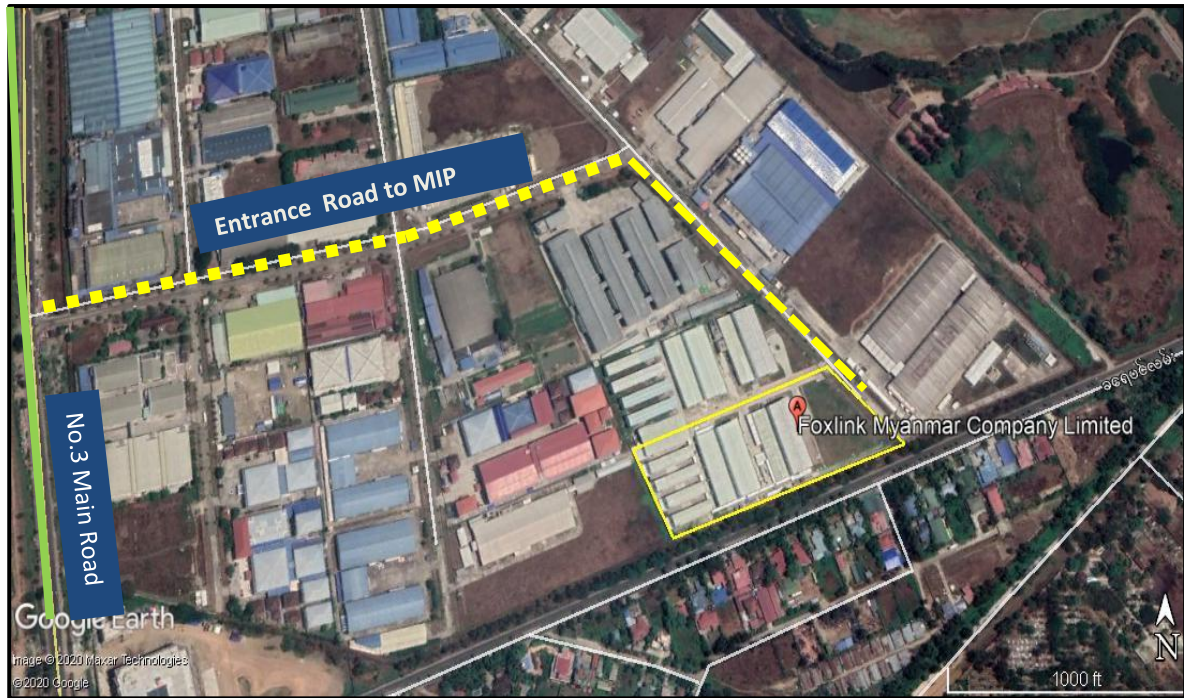
Figure 3-2 Access Road to the Proposed Project
