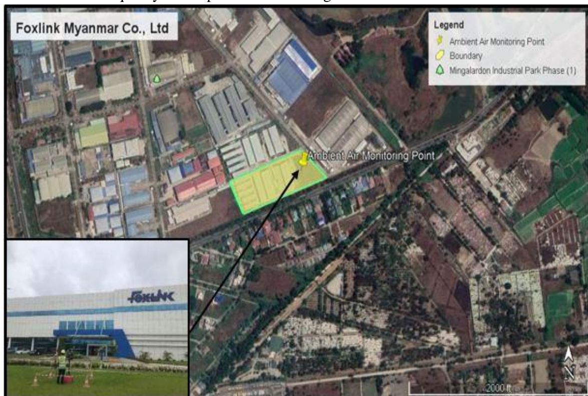
Figure 4-1 Ambient Air Quality Measurement Point
