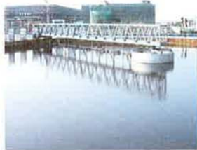
Full-bridge Peripheral Drive Mud Scraper (24000mm)
