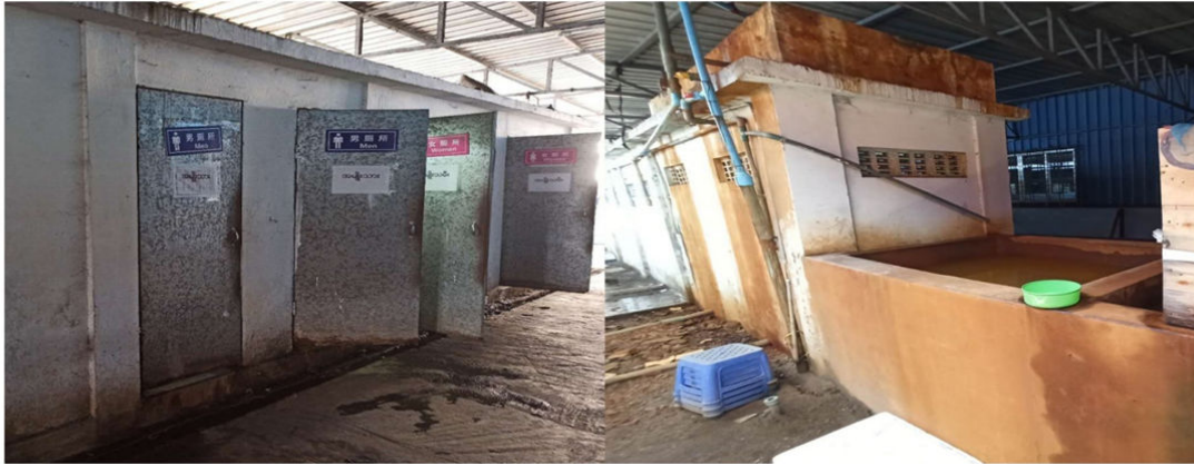
Figure 6-3 Toilet Facilities in factory at Myanmar Yarn & Fabric Technology Factory
