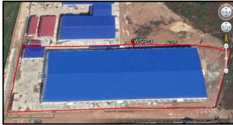
Figure 4-11 Location of Water Sampling Point (Wastewater Quality)
