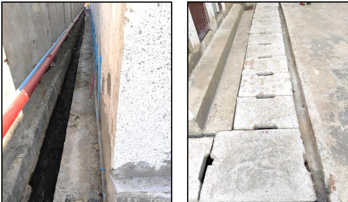
Figure 2-32 Drain Channel inside the Factory
