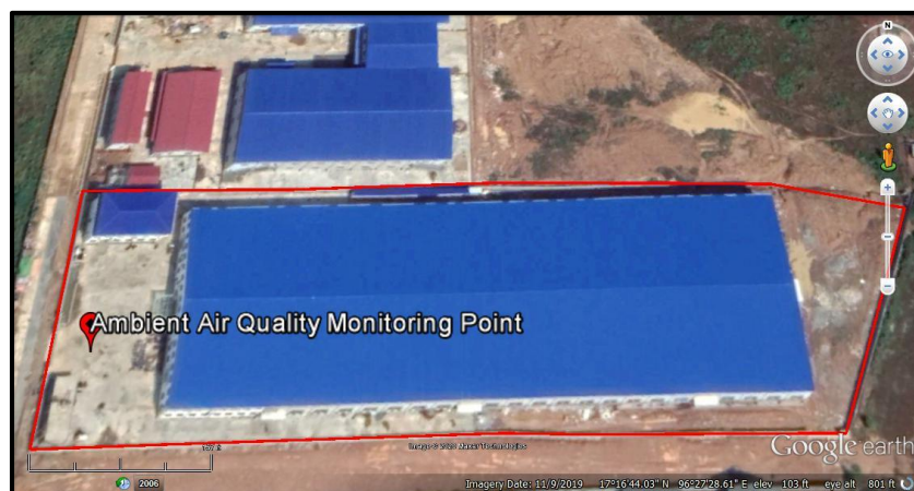
Figure 4-2 Location of Measuring Ambient Air Quality
