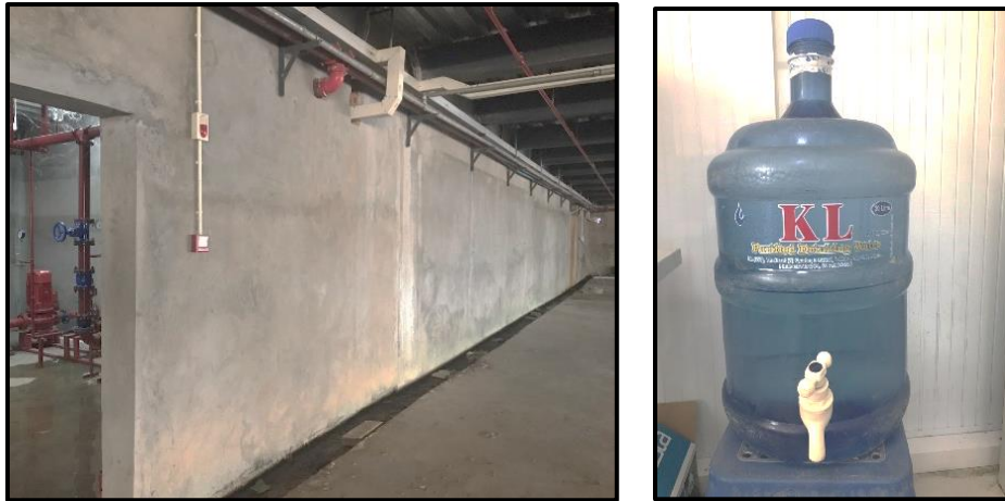
Figure 2-27 Water Storage Tank and KL Drinking Water
