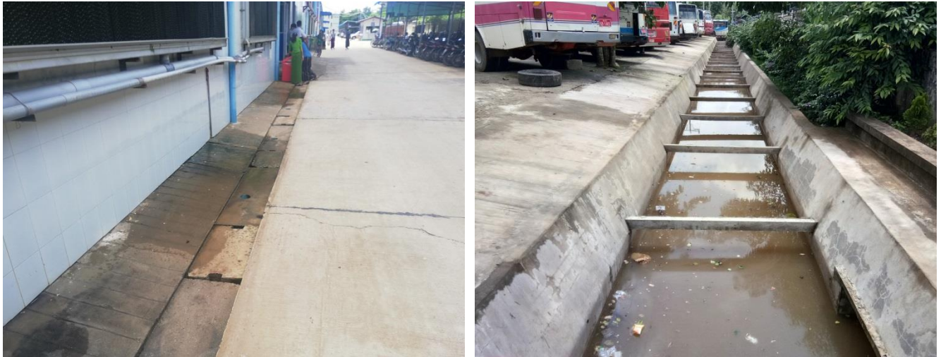
Figure 3-17 Rainwater drainage in factory compound
