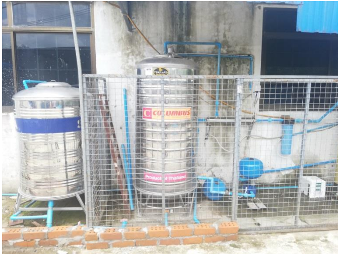
Figure 3-10 Water storage Tank and Overhead Tank
