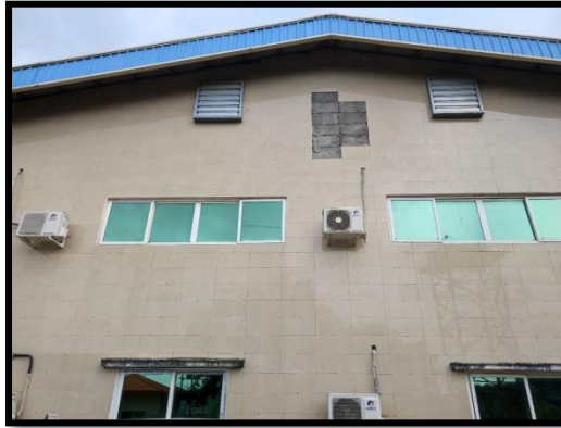
Figure 3-17 Photos of Ventilation
