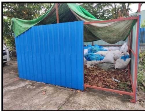
Figure 3-16 Photos of Garbage Room and Bin
