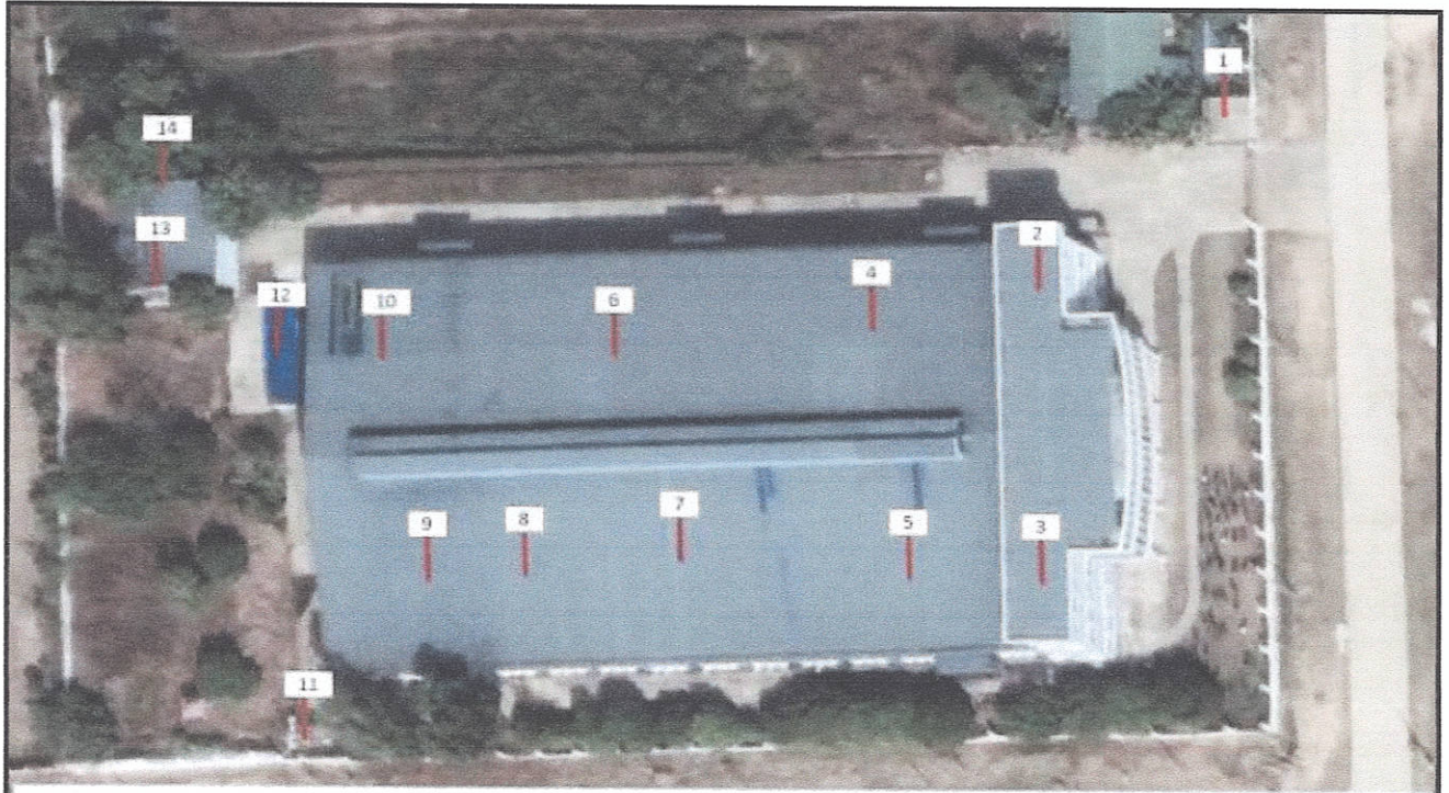
1. Security Gate 2. Clinic & Child Care 3. Office 4. Warehouse 5. Cutting Area 6. Canteen 7. Sewing Line Area 8. Quality Control 9. Sewing Machine Area 10. Finished Products & Packaging 11. Transformer 12. Toilets 13. Waste Storage Area 14. Water Pump
