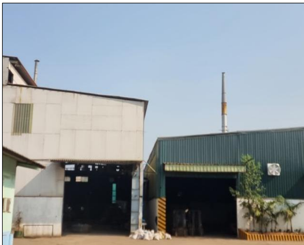
Figure 3.11 Chimney's Current Condition (as of February 2024)
