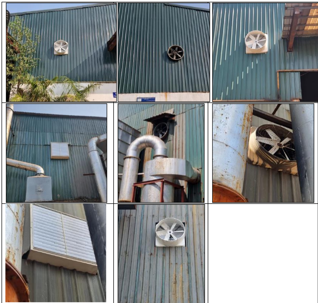
Figure 7.6 Exhaust Fan Installation Condition
