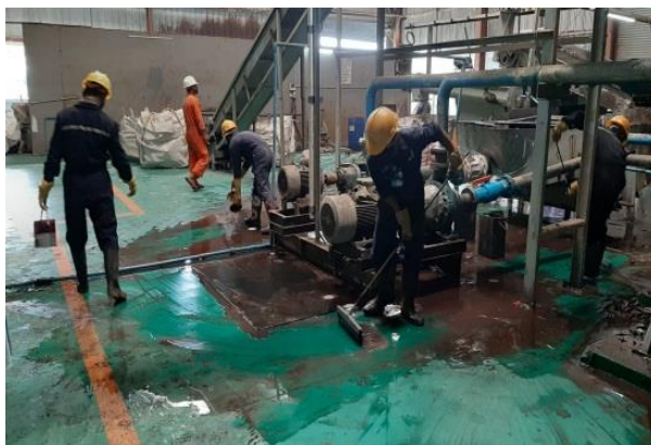
Figure 3.33 Image of Epoxy Lined Floor Cleaning
