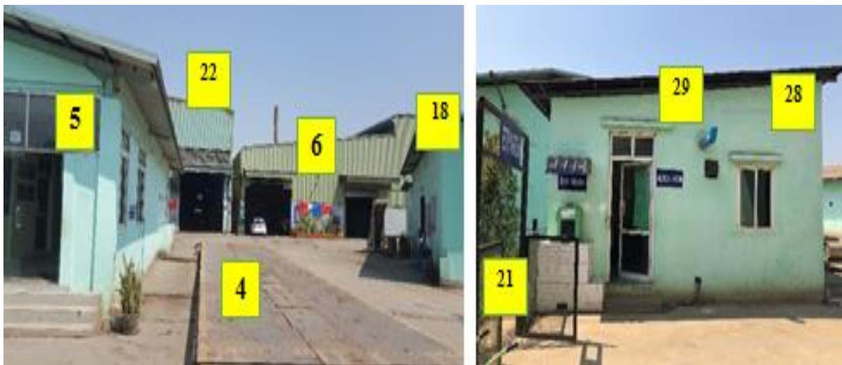
Figure 3.7 Photos of Factory Buildings
