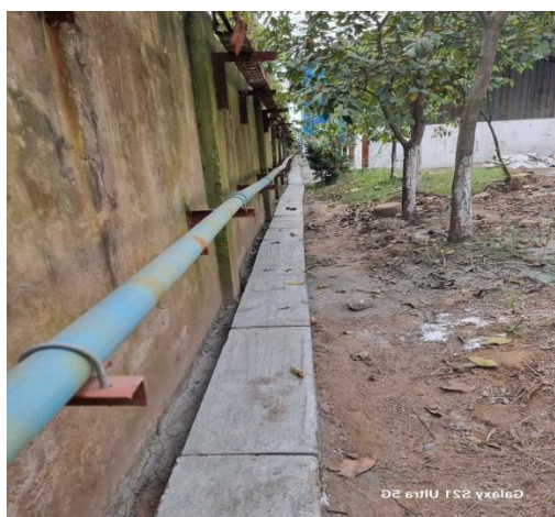
Factory Drainage Channel
