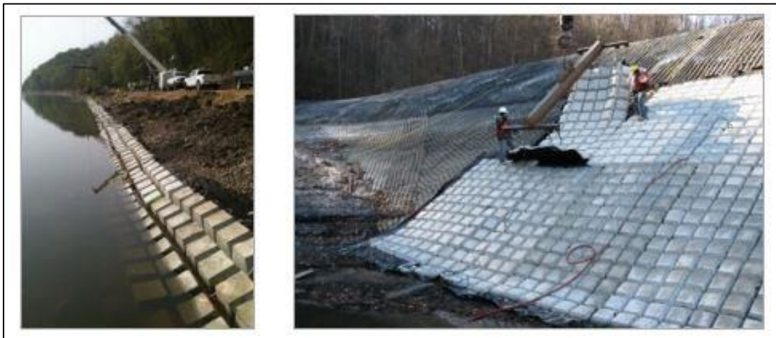
Figure 3-87 Example Pre-Cast Concrete Block Mattress with Geotextile
