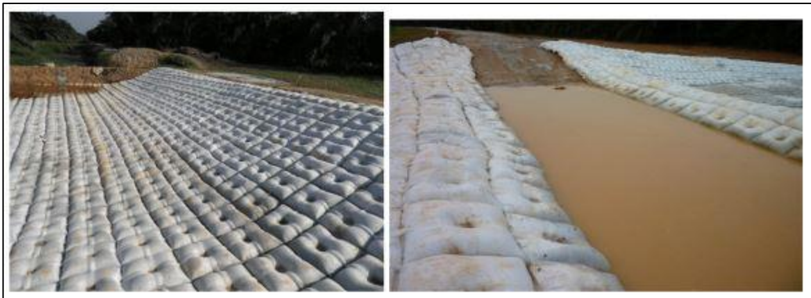
Figure 3-89 Example Concrete Flexible Mattress System
