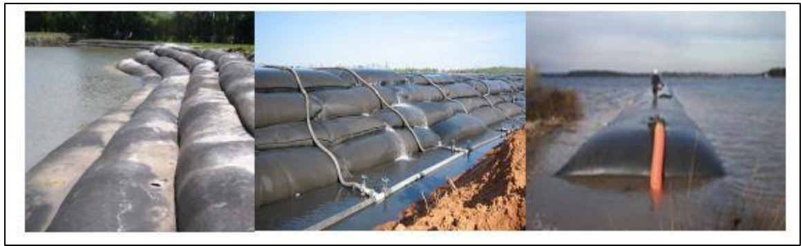
Figure 3-93 Examples of Geotube Systems
