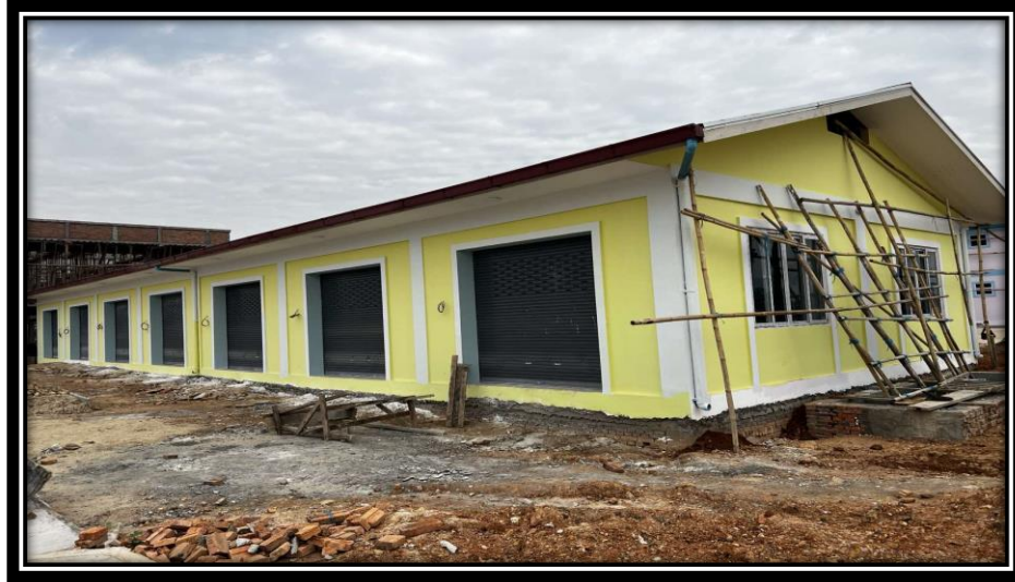
Figure 4.11 8 units & 7 Units One Storied Mini Bus Gate
