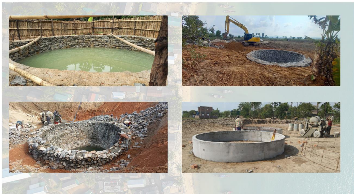
Figure 4.34 Images of 20 ft wide ground water well
