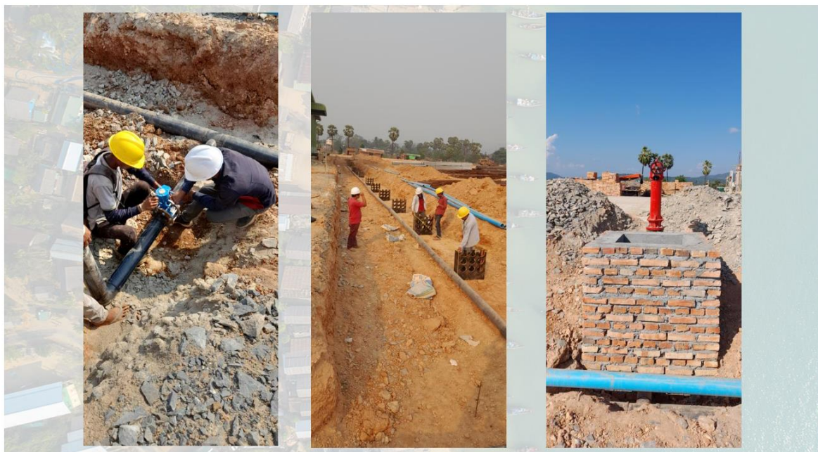
Figure 8.6 Fire Hydrants installation
