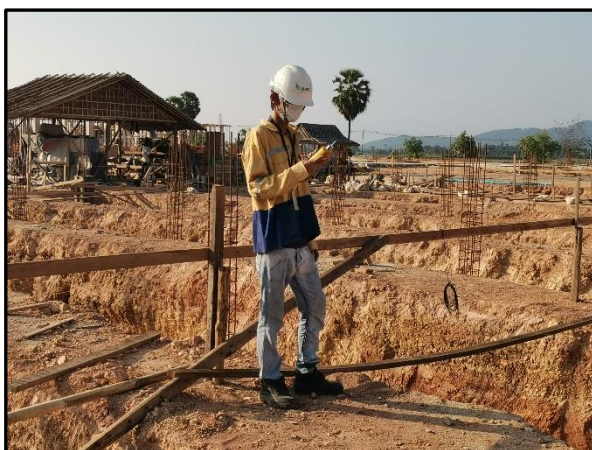
Odor Measuring at Point 3 (Near the Center of the Project Site) in the dry season
