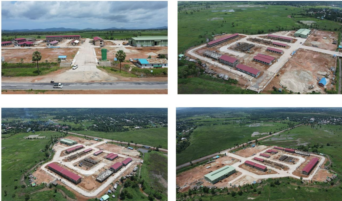
Figure 4.5 Ariel pictures of Project Site
