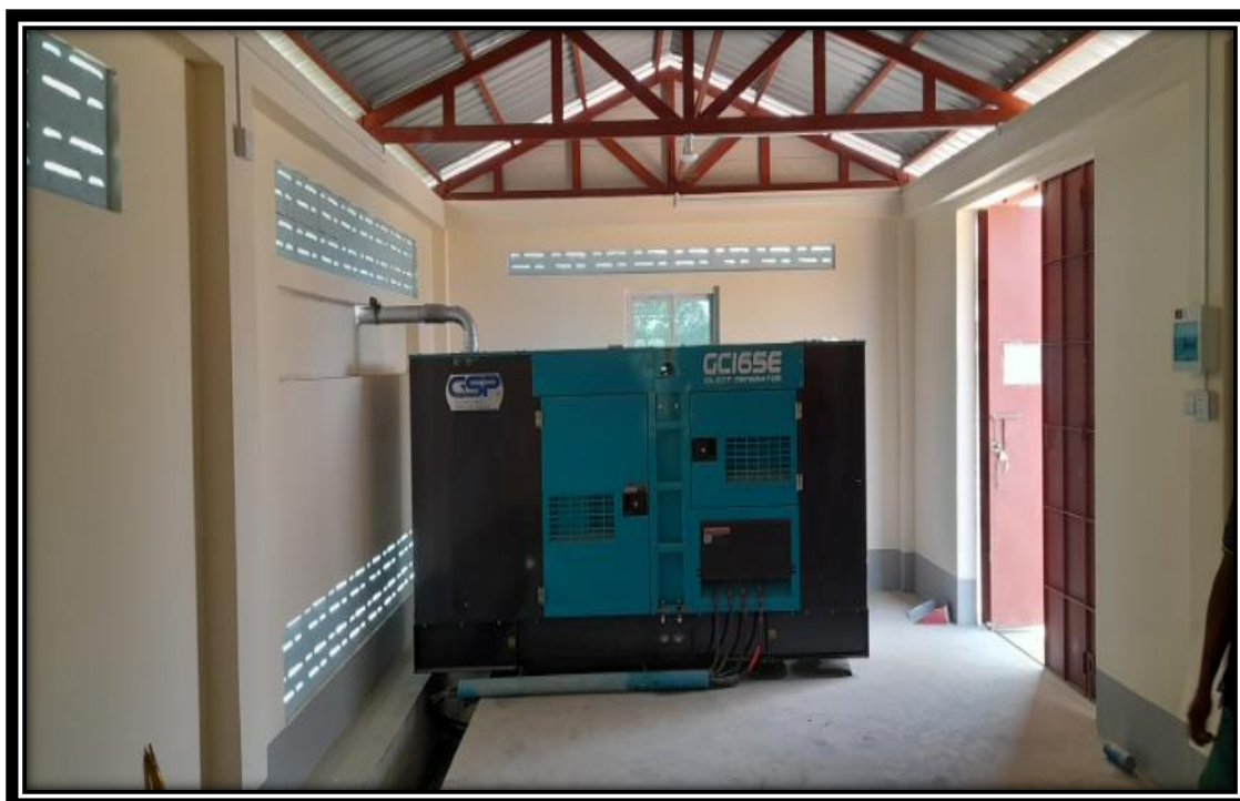
Figure 4.22 Infrastructure M&E work
