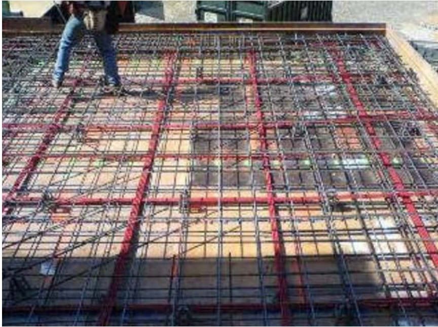
Figure 3.6-1 Construction of Post-Tensioned Slab
