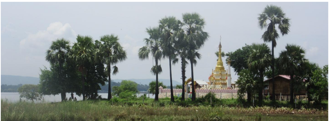
Figure 2.13. View of Tae` Nan Thar Phaya very closed with Proposed Development Site
