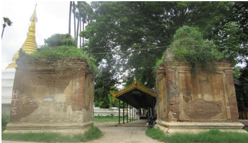
Figure 3.11. View of the Entrance Gate of MAHAVIJAYARAMSI Pahtodawgyi Pagoda
