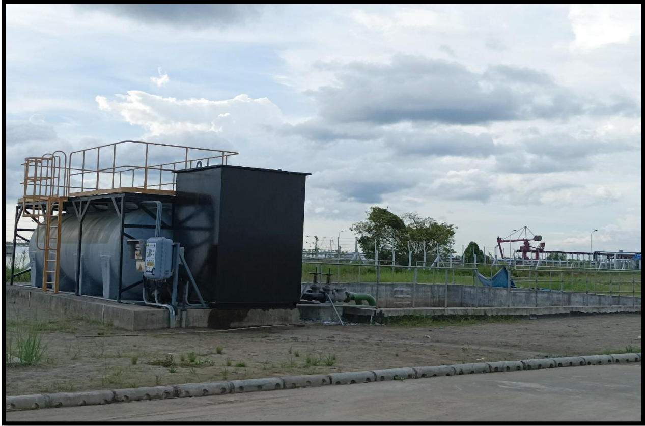
Photo 6: Oily water separator, networks and pit installation
