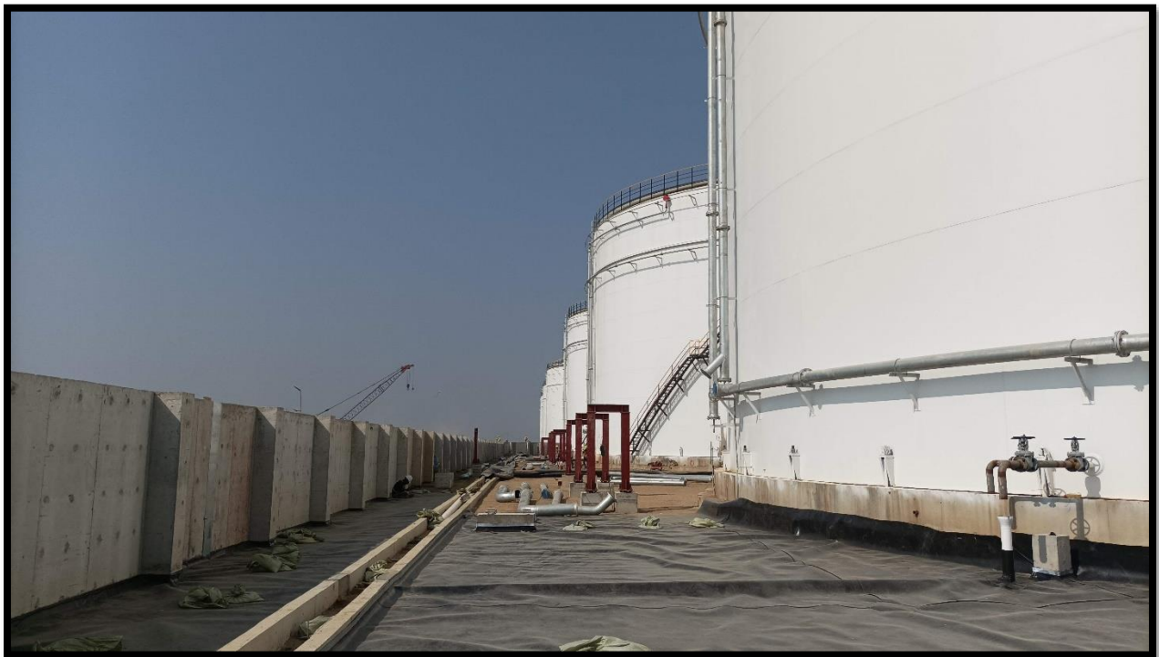
Photo 5: Installation of HDPE membrane inside the Diesel Tank Farms
