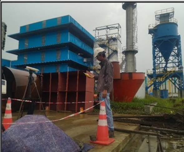
Between Feed Mill & Biomass Power Plant (OP3) Wet Season
