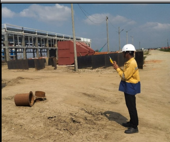
Between Feed Mill & Biomass Power Plant (OP3) Dry Season
