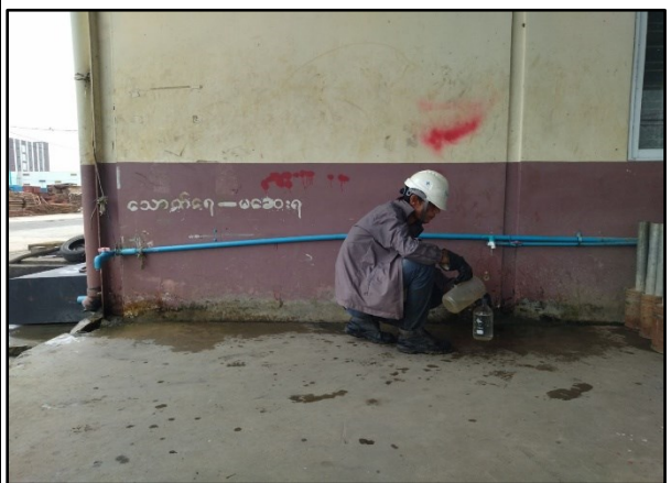
Drinking Water Treatment Plant (P 1) Wet Season
