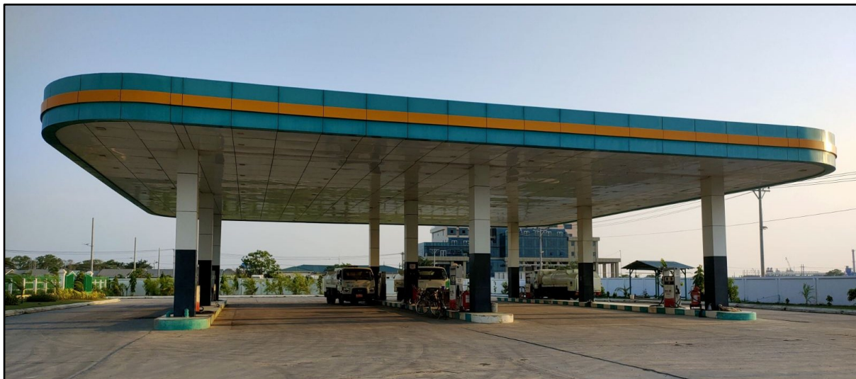
Photo (4.14) Fuel Storage Tank Terminal
