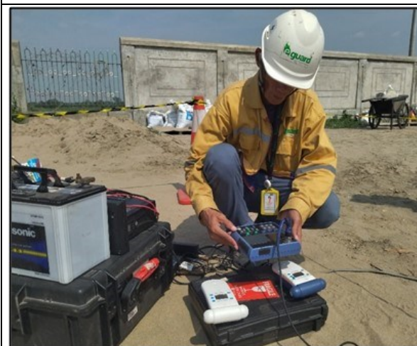
Between Feed Mill & Biomass Power Plant (V 3) Dry Season
