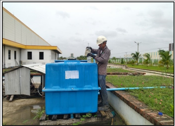
Processing Plant and Cold Storage (Tube well) (WP 7 GW) (Wet Season)
