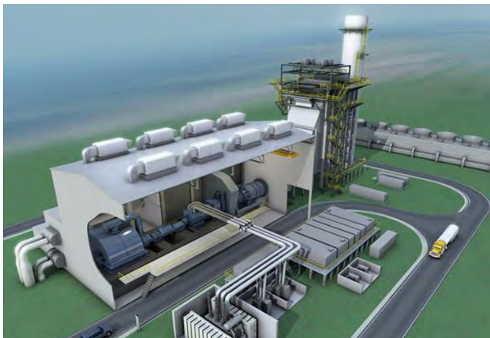
Figure 12. 1 Generic Image of a CCGT power plant with one Gas Turbine Building
