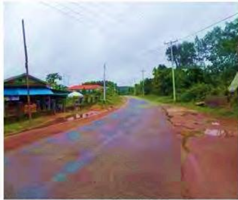
Paved Road south east of the Site
