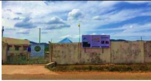
Fencing around the proposed CCGT site, with signage regarding the Project
