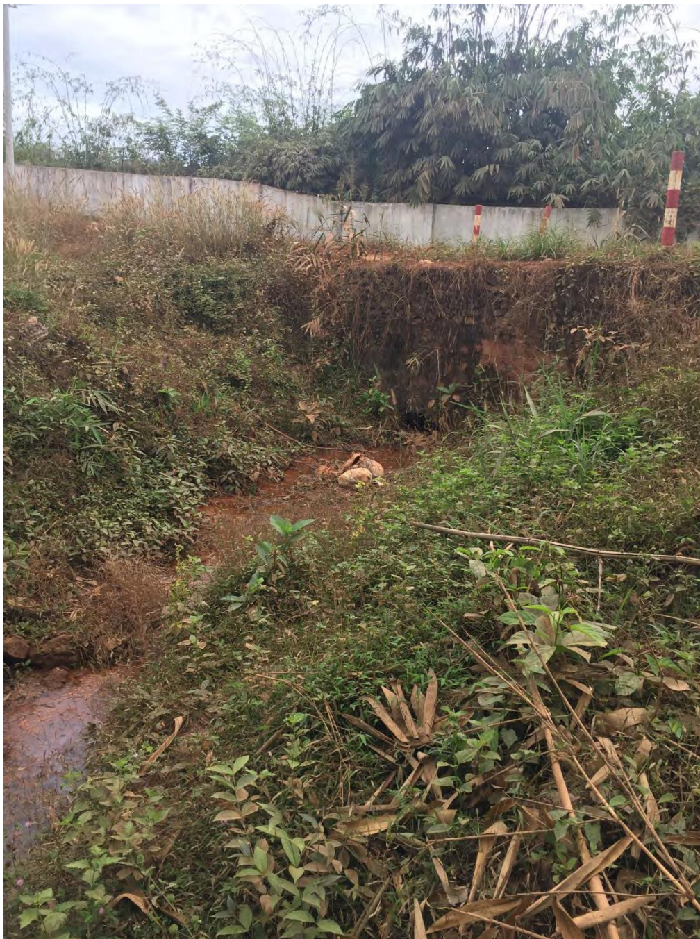
Figure 4. 12 Wastewater Discharge Point
