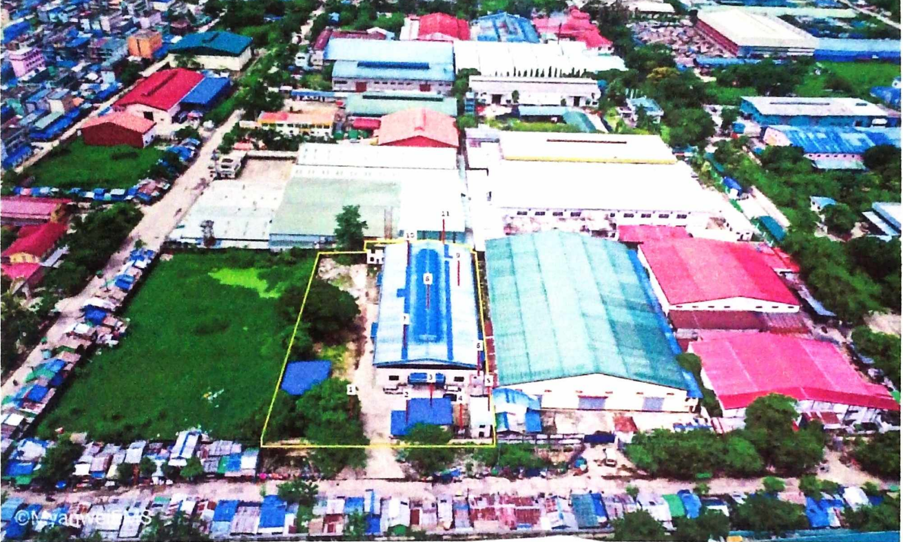
1.Security Gate 2.Generator Room 3.Canteen 4.Transformer 5.Dormitory 6.Overhead Tank 7.Office 8.Sewing and QC Area 9.Cutting and Ironing Area 10.Warehouse 11.Toilets
