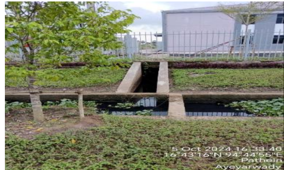
Drainage Outlet to Central Drain
