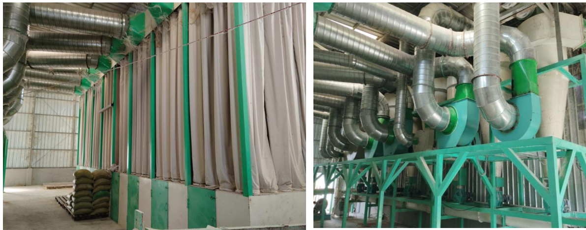
Figure 2-16 Air Pollution Control Measures
