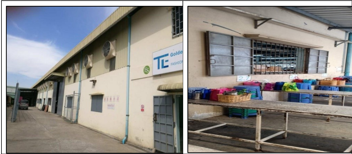
Figure 4-21: Photo of Ventilation
