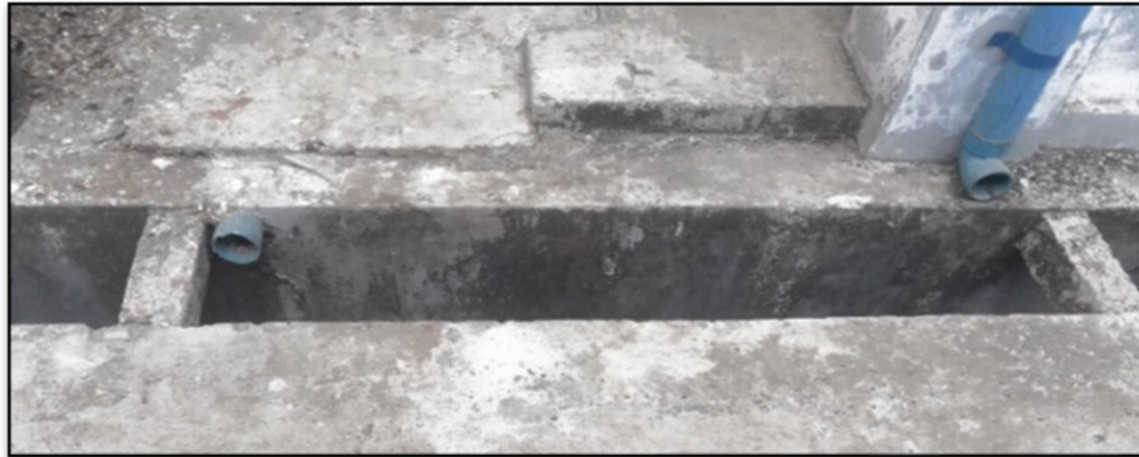
Figure 4-19: Photo of Drainage
