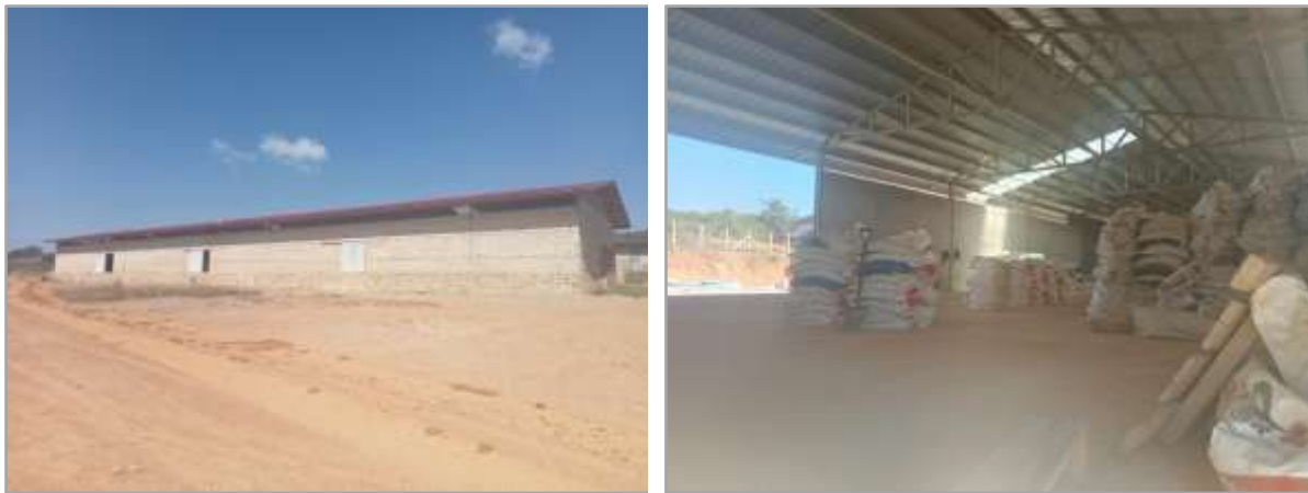
Figure 4.8 Warehouse in Lead Washing Plant
